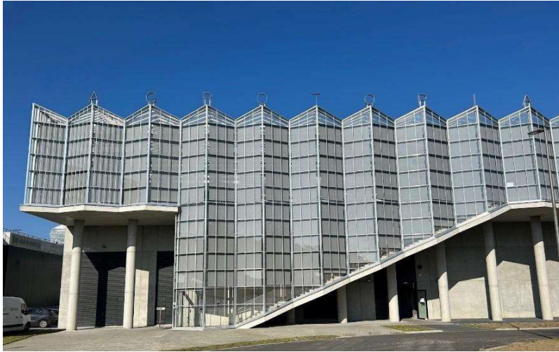
Figure 4.1- a) Agrotopia Rooftop Greenhouse and Façade (photographed by author during site visit)
