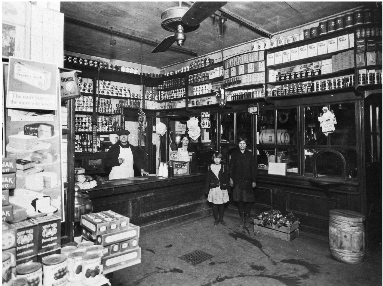
Fig. 3: A typical turn-of-the-century dry-goods grocer. Goods were stacked behind a counter or in a storeroom, only to be handled by the shopkeeper. Pictured is a store in East St. Louis, Ill. in 1914. (Shorpy Historic Photo Archive)
