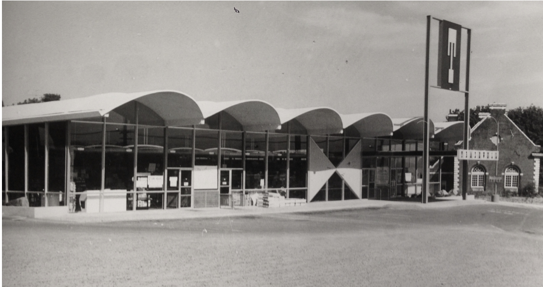
Fig 34: Columbia City Tradewell pictured shortly after opening. Architect Welton Beckett, whose early career included drive-in markets in Seattle, designed three award-winning experimental concrete structures for the chain. They did not catch on, and Beckett's later designs for Tradewell were more conventional. ( American Builder , 1958)
