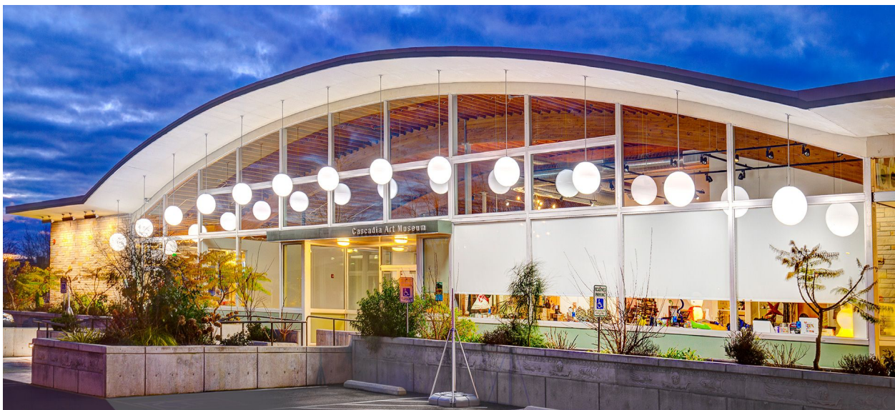
Fig. 47: The remodel process left much of the character-defining features, such as the glue-laminate beams, curtain wall mullion pattern, and brick veneer, substantially intact, while updating mechanical systems to meet modern needs. New hardscaping buffers the building from the parking lot. (Tom Marks, Seattle Daily Journal of Commerce )
