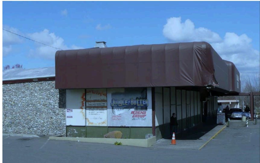
Fig. 35: Columbia Plaza in 2008. Much of the exterior glazing was obscured with solid panels, and the expressive roof overhangs were truncated to accommodate the awning. These modifications challenged the historical integrity of the building. (BOLA Architects + Planners)
