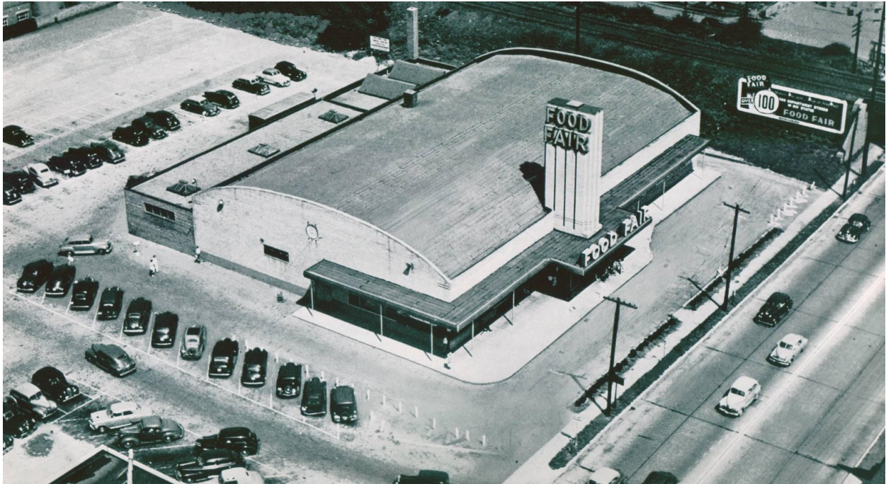
Figure 9: Food Fair Market in Collingswood, N.J., circa 1945. In the first decade after World War II, the pace of supermarket construction exploded, and stores featured a more utilitarian design that was easily replicated at scale. The growing popularity of the Modern Movement meant that these simple, unadorned forms were in vogue. (Pleasant Family Shopping)
