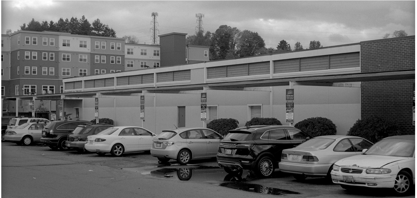
Fig. 41: UGM administrative offices in 2018. Like many of the other case studies, much of the exterior glazing is now obscured. In 2011, some of the ‘five acres of parking’ was given over to a new emergency homeless shelter. (Author)
