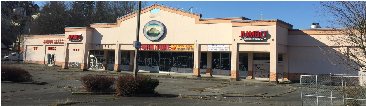
Fig. 37: Rainier Mall pictured in 2019, now vacant for over two years. Though the façade bears little resemblance to the original appearance, the iconic arched roofline is obscured but intact. (Author)
