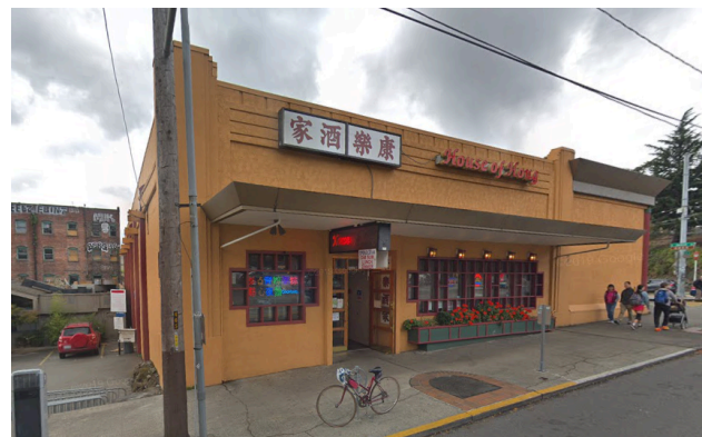
Fig. 22: House of Hong, in the International District, is a rare standing example of a prewar supermarket in the Seattle area, built as a Safeway in 1940. (Google Street View, 2018)
