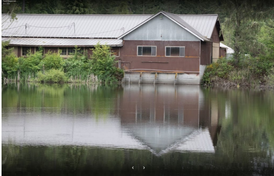
Figure 43. Derelict Warehouse & Pond
