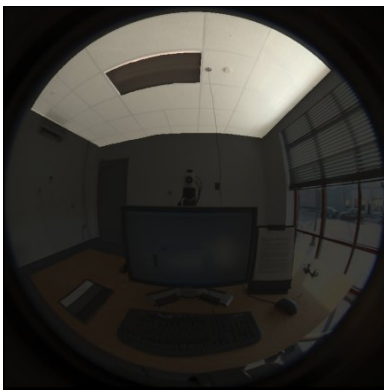
Figure 48 – Mask 14 (X14) encompasses the ceiling plane excluding the electric light fixture
