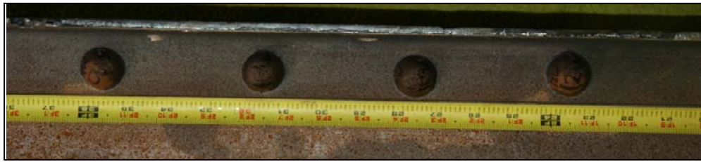
(a) West Channel Prior to Testing
