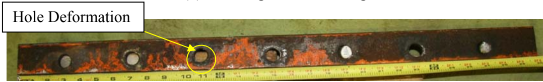
(c) East Channel After Testing
