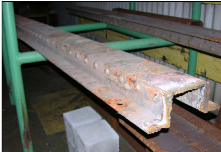
Figure 3.6 Original Guardrail Specimen
