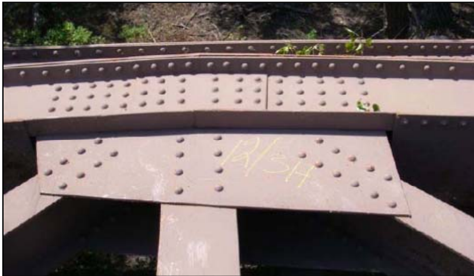
Figure 3.5 Joint U3 from Bridge 1
