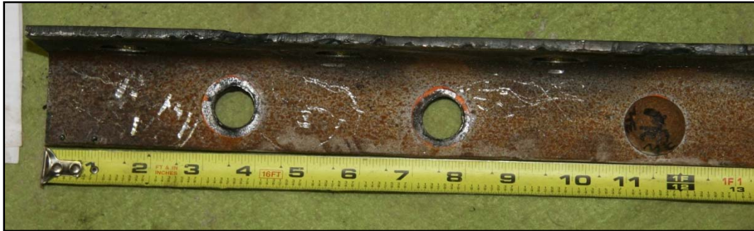
(b) Top of Channel
