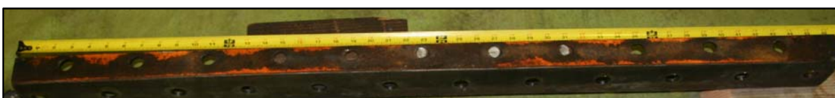
(c) West Channel After Testing
