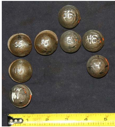
(a) All Fractured Rivets
