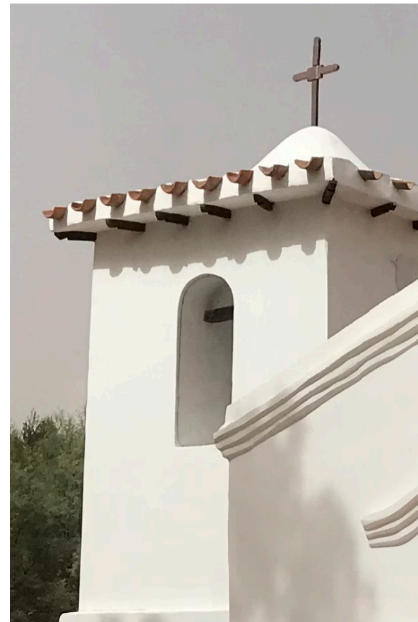
Fig. 32: San Pedro Church bell tower, Dec. 2019.
