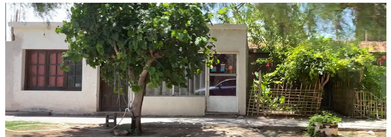
Figs. 64-66 (top right to bottom): Modifications from standard to resident-reflective social housing, December 2023.
