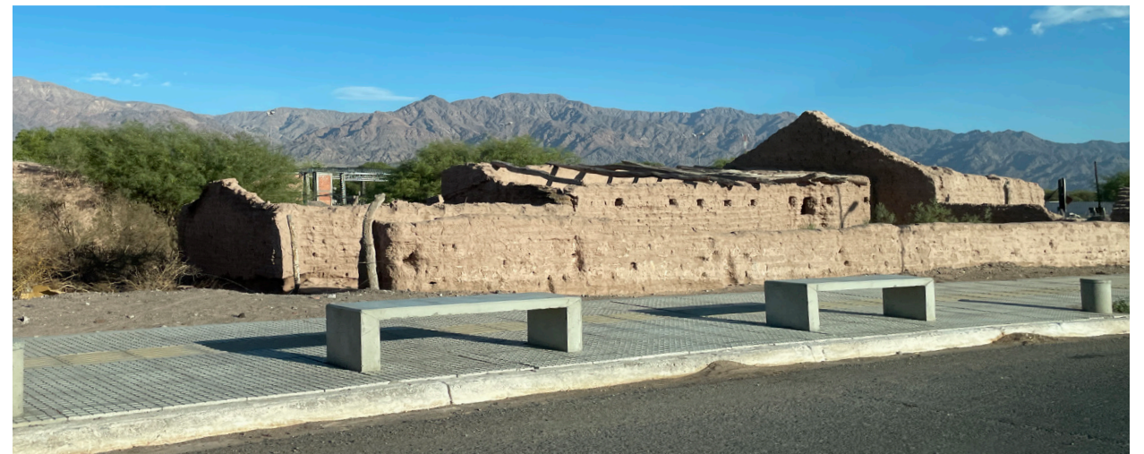
Fig. 26: Abandoned adobe building, December 2023.
