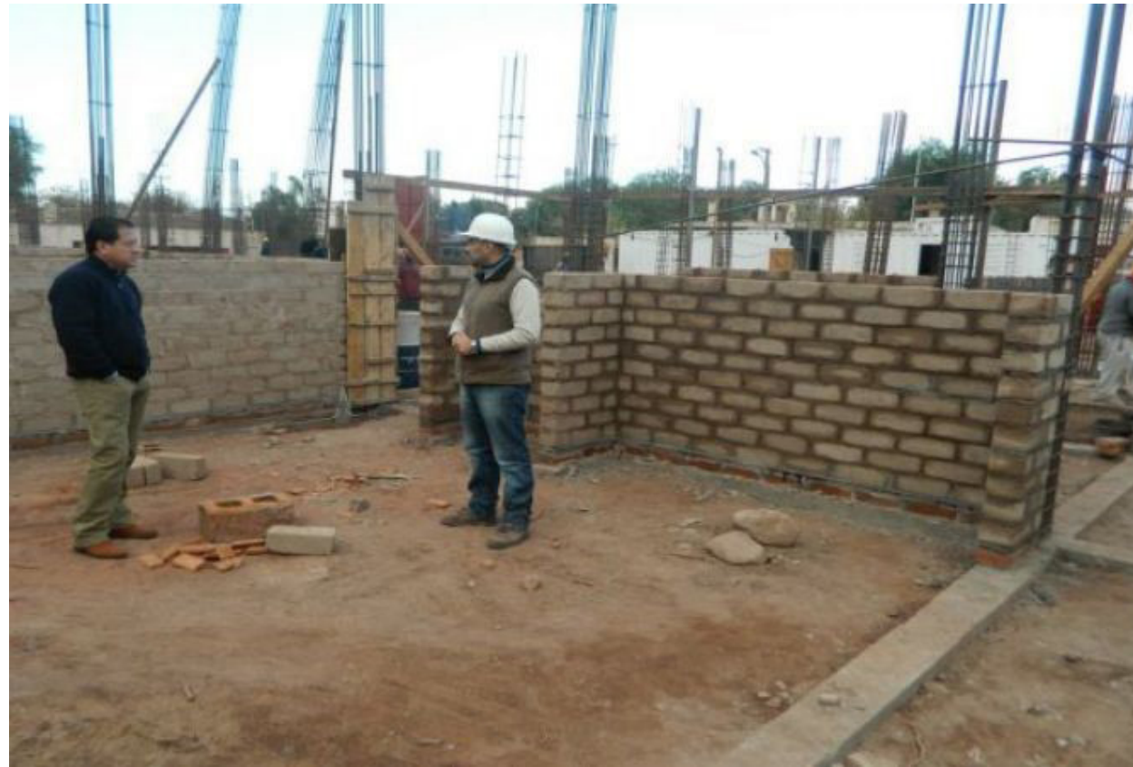
Fig. 15: The Esquiú Newspaper, Exposed CEB Masonry and Rebar Frame, November 2012.
