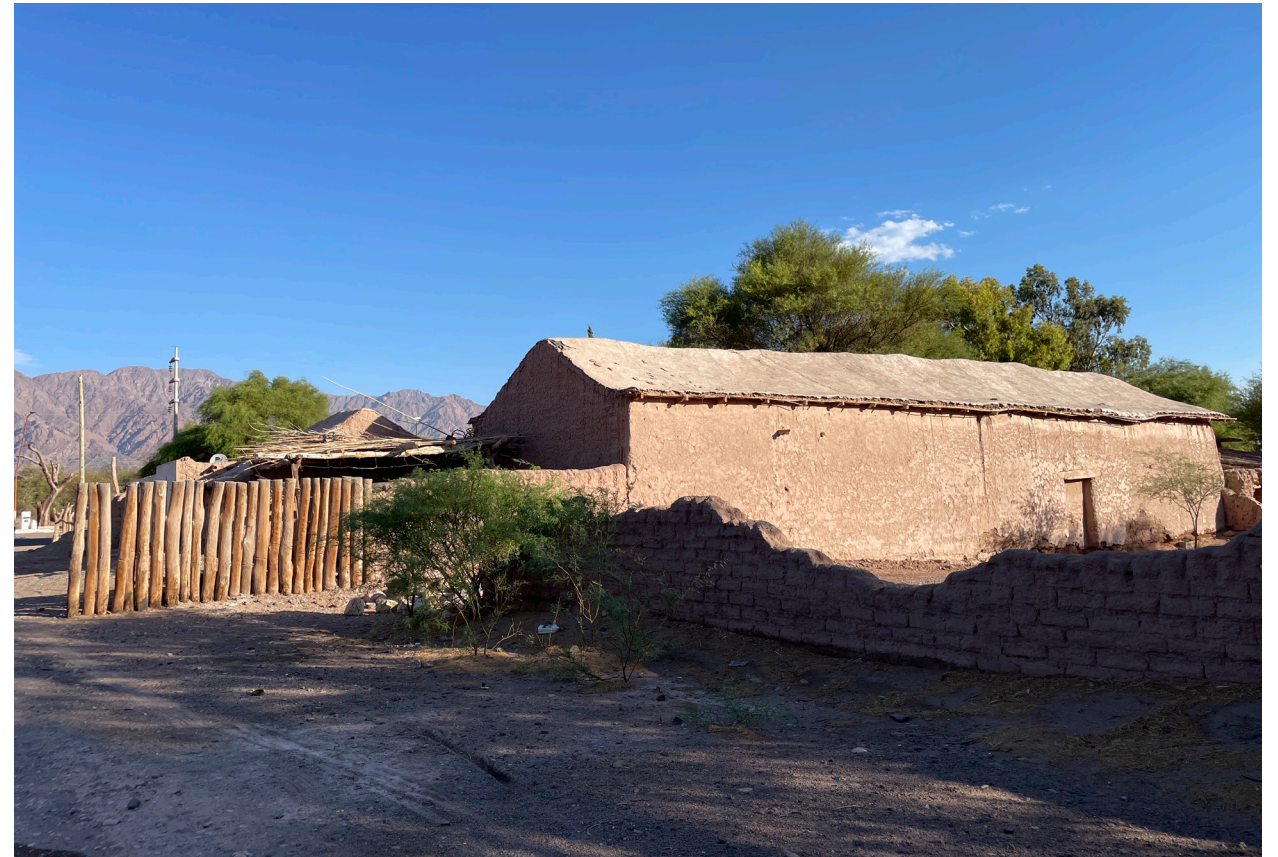
Fig. 25: Comandancia de Armas building, December 2023.
