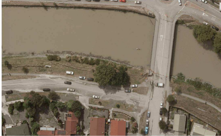
Figure 1.7: Avondale Road Bridge after the Christchurch event. Lateral spreading cracks are visible near the southern approach and along the river bank (LINZ, 2011).
