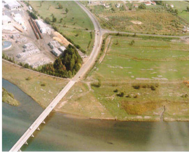
Figure 1.2: Northern approach to Landing Road Bridge two days after the Edgecumbe event. Ejected sand is visible on the ground surface (Berrill and Yasuda, 2002).
