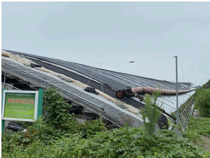
Figure 1.8 Exterior of a passive solar greenhouse
