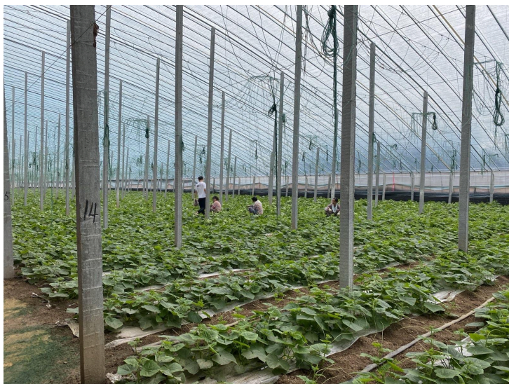
Figure 1.9 Interior with concrete columns
