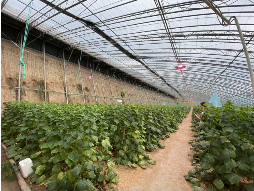
Figure 1.12 Interior of a steel truss PSG with supplemental lighting.
