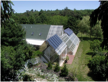
Figure 1.3 Cape Cod Ark, 2004 (The Green Center)
