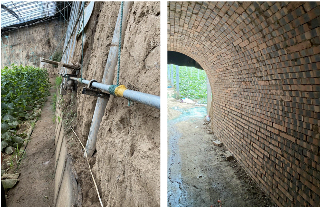
Figure 1.11 Vent control system with rods and ropes (left). Entrance (right).
