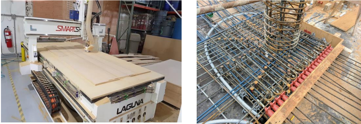
Figure 4.11. Installed slab formwork fabricated using the CNC machine
