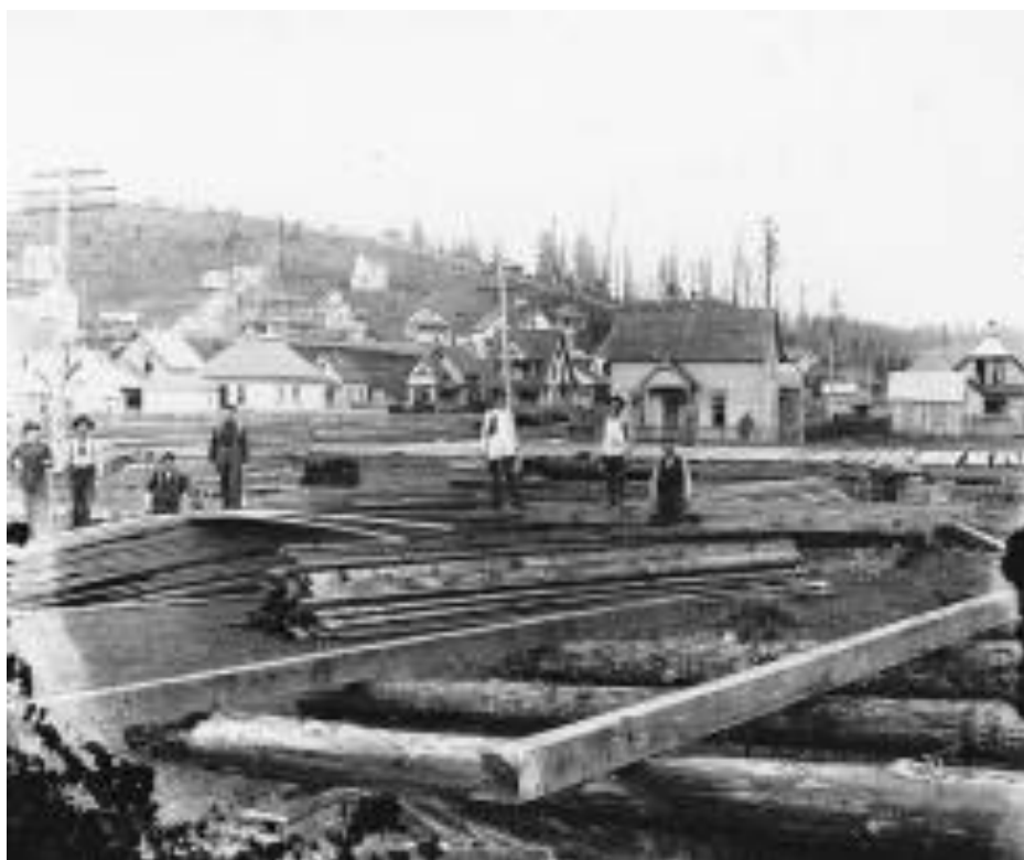
Figure 3-11. Construction of streets in Hoquiam c. 1908, using planking necessary to keep them out of reach of high tides. (University of Washington Libraries, Special Collections, Order Number WAS0195, Negative Number UW348)
