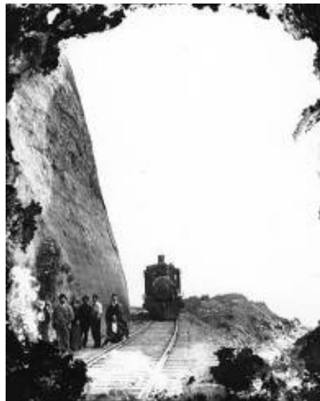
Figure 3-16. First engine to run on the new Northern Pacific railroad line connecting Hoquiam to Moclips in 1909. The rail was laid on fill at base of steep bluff west of Hoquiam. (University of Washington Libraries, Special Collections, Order Number WAS1060)
