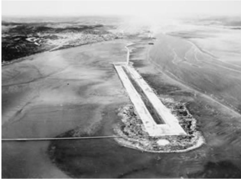
Figure 3-21. Expansion of Moon Island Airport by U. S. Army Air Corps as part of World War II West Coast defense. In foreground, note railroad trestle, which was used to transport materials from the north shore (just outside of the frame to the left) in the construction effort. Piling from this trestle remains in the wildlife refuge, and the eastern access point to the current gathering grounds is near these pilings where they reach the north shore. (Port of Grays Harbor, http://portofgraysharbor.com/about/history/index.php )
