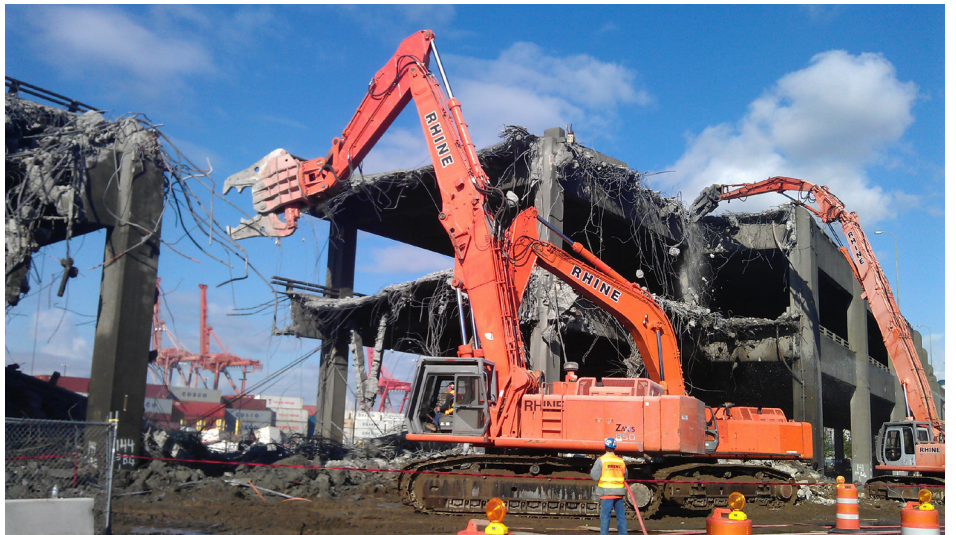
83: Photo: Alaskan Way Viaduct Demolition
