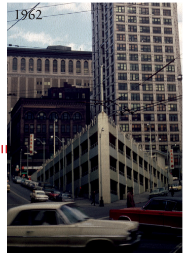
71: Photo: Sinking Ship Parking Garage
