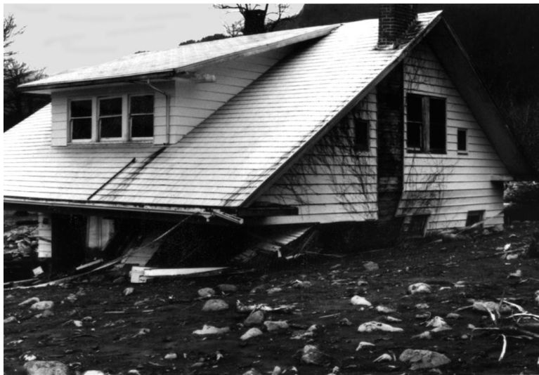
Figure A2.5.1. The 08 Feb. 1996 West Dodson, Oregon, debris flow carried away the furnishings of this home while leaving it on its foundations. Image: Iverson et al. (1997).
