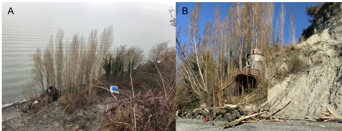
Figure 6.33. An actively occupied encampment ( A ) that is sitting on the deposit of a large debris fall that occurred in 2013 ( B ). Note the structure in both images for reference. Photos: J. Wartman and W. Pollock.
