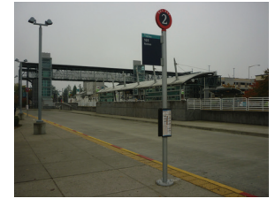
Figure 50 Kent Station Rail Stop
