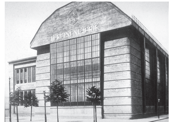
Figure 8 AEG Turbine Factory - Behrens
