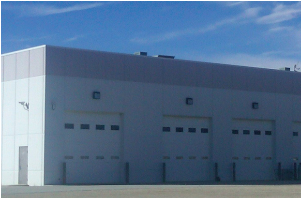
Figure 2 Generic Manufacturing Facility Exterior
