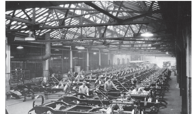
Figure 6 Packard Building - Kahn
