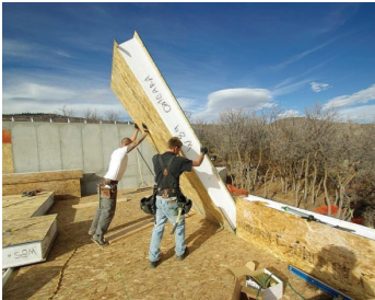
Figure 18 Prefabricated SIPS Panel
