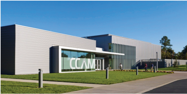
Figure 26 CCAM Exterior View
