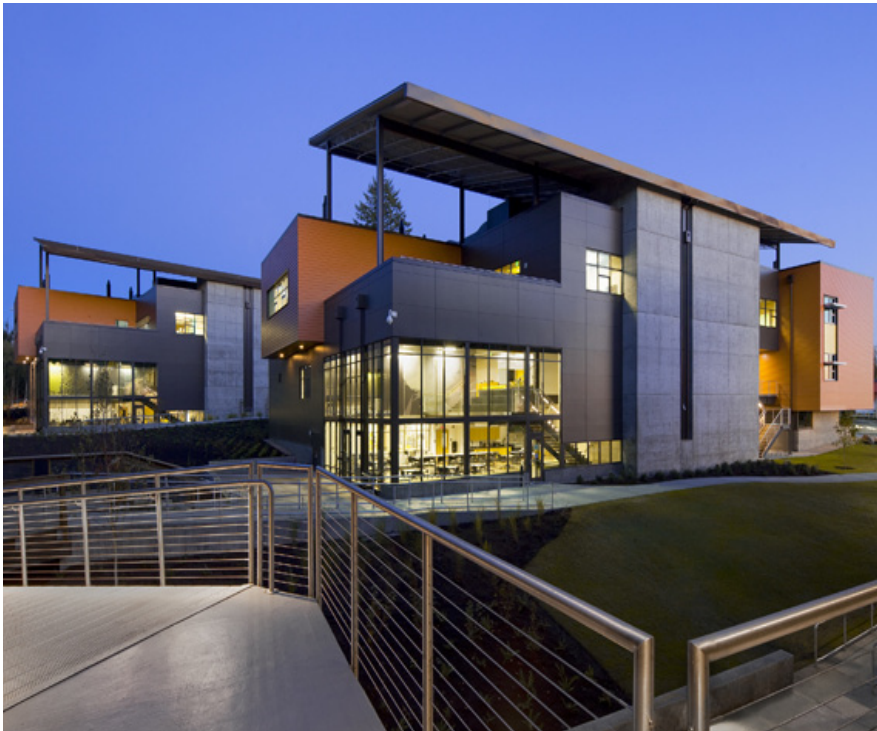
Figure 38: Marysville Getchell High School is comprised of four identical buildings that house autonomous learning communities.
