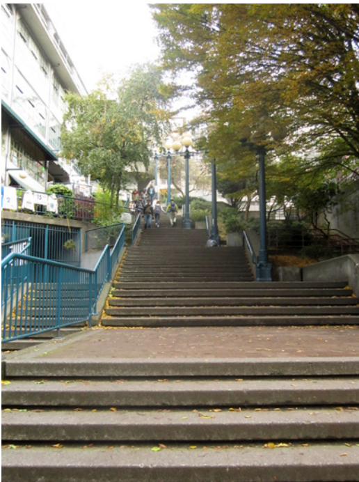
East of the site - Pike Street Hill Climb
