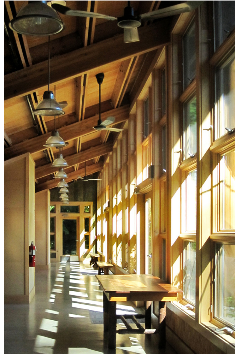
Figure 33: IslandWood - The solar lobby of the learning studios acts as a heat sink for the building.
