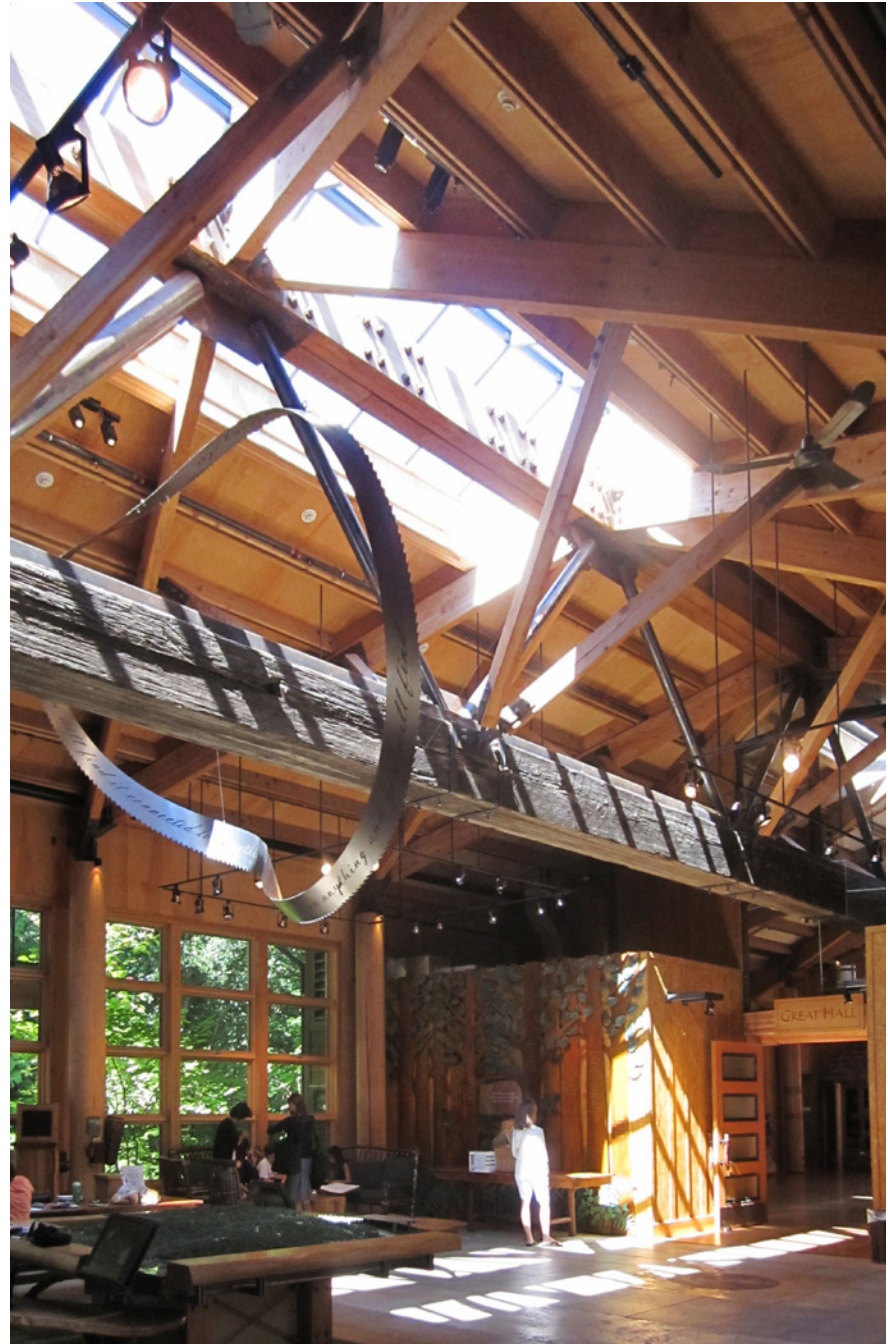
Figure 34: IslandWood - The 92-foot, 120-year-old salvaged wood beam that was found abandoned in a field is the main design element in the Welcome Center.
