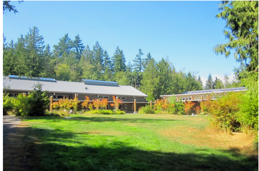
Figure 29: IslandWood - View of the dining hall and learning studios buildings and adjoining solar meadow
