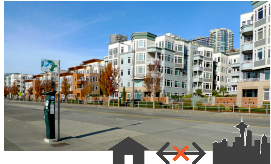
Figure 56: Disconnect between the waterfront and the city
