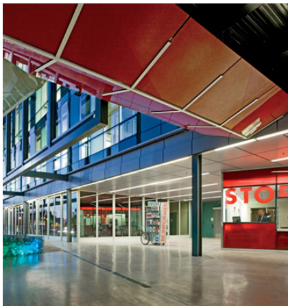
Figure 2.41 Tempe Transportation Center- Entrance view
