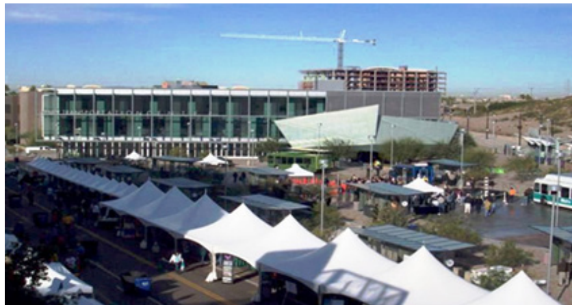
Figure 2.42 Tempe Transportation Center- Bird eye view
