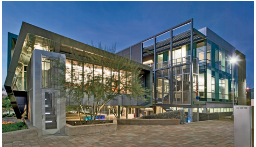
Figure 2.40 Tempe Transportation Center- Exterior view at night
