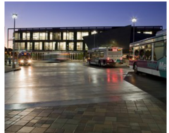
Figure 2.43 Tempe Transportation Center- Transit plaza
