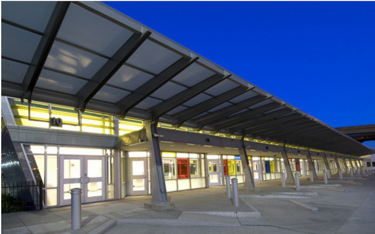
Figure 2.19 Gateway Multimodal Transportation Center - Entry canopy
