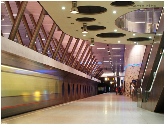
Figure 2.34 Metro Stations- Wilhelminaplein station, Rotterdam
