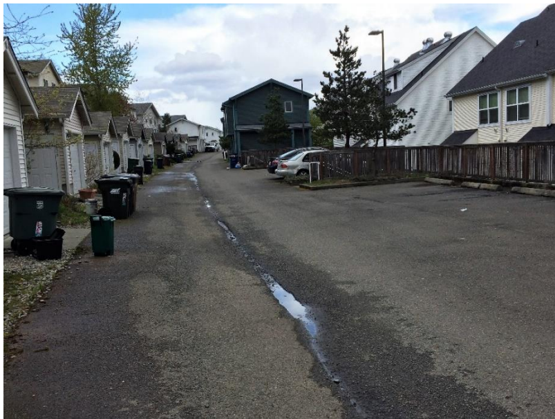
Figure 4.8. Alley between 39th Ave S and Rockery Dr S (source: Author).
