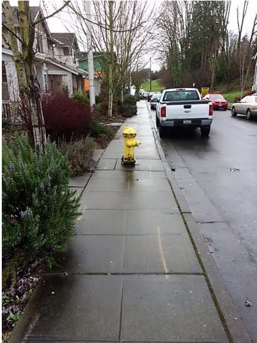
Figure 4.9. Fire hydrant in sidewalk, creating a path obstruction (source: Author).
