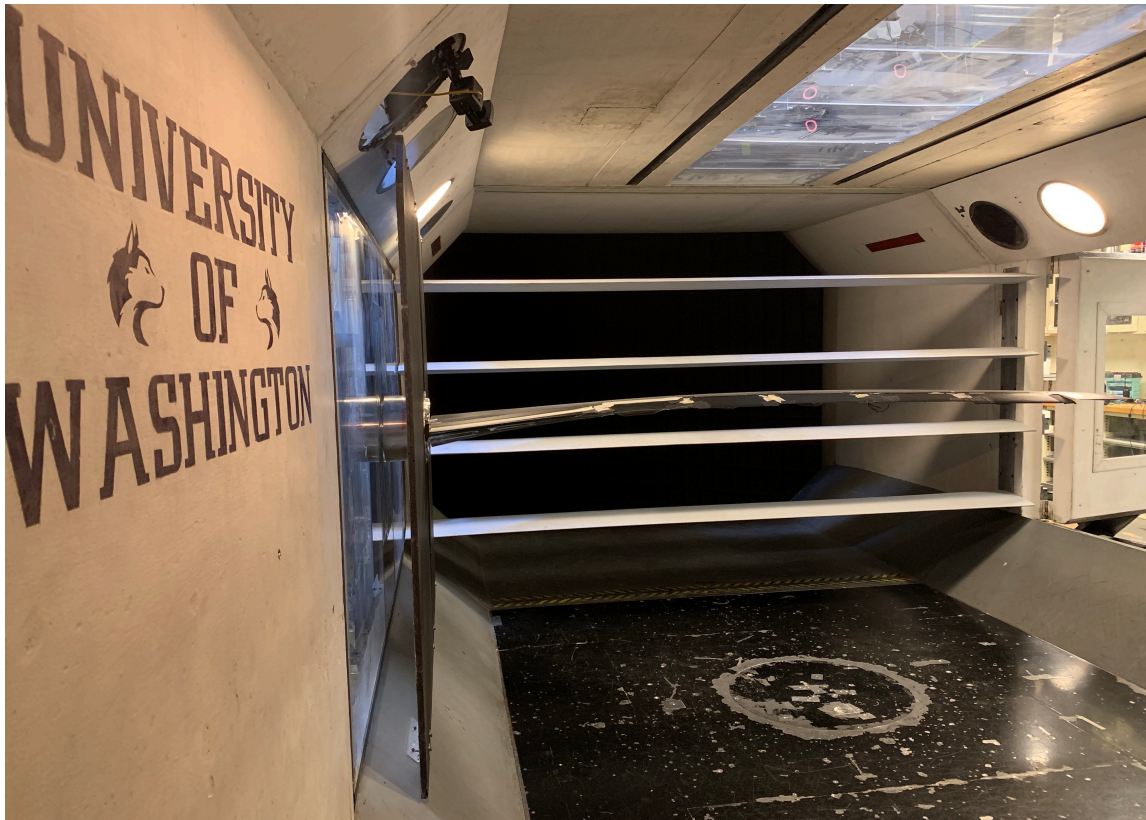
Figure 53: Installed Wing IV and gust generator vanes showing splitter plate offset
