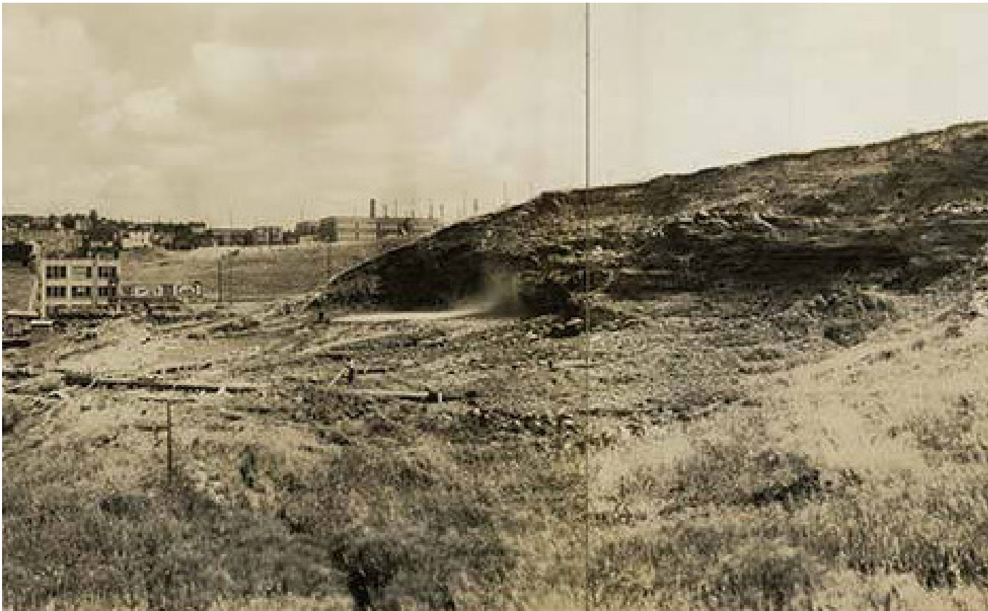
Figure 42. Beacon Hill regrading, Seattle, ca 1923 (Museum of History & Industry Collection, MOHAI, Lockheed Shipbuilding & Construction Company Photographs and Publications, 1988.13.7.2.58)
