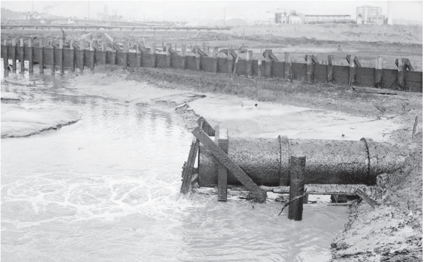
Figure 62. Pipe discharging sewage into the Duwamish River at Diagonal Way, ca. 1938 (Museum of History & Industry Collection , 1983.10.10091)
