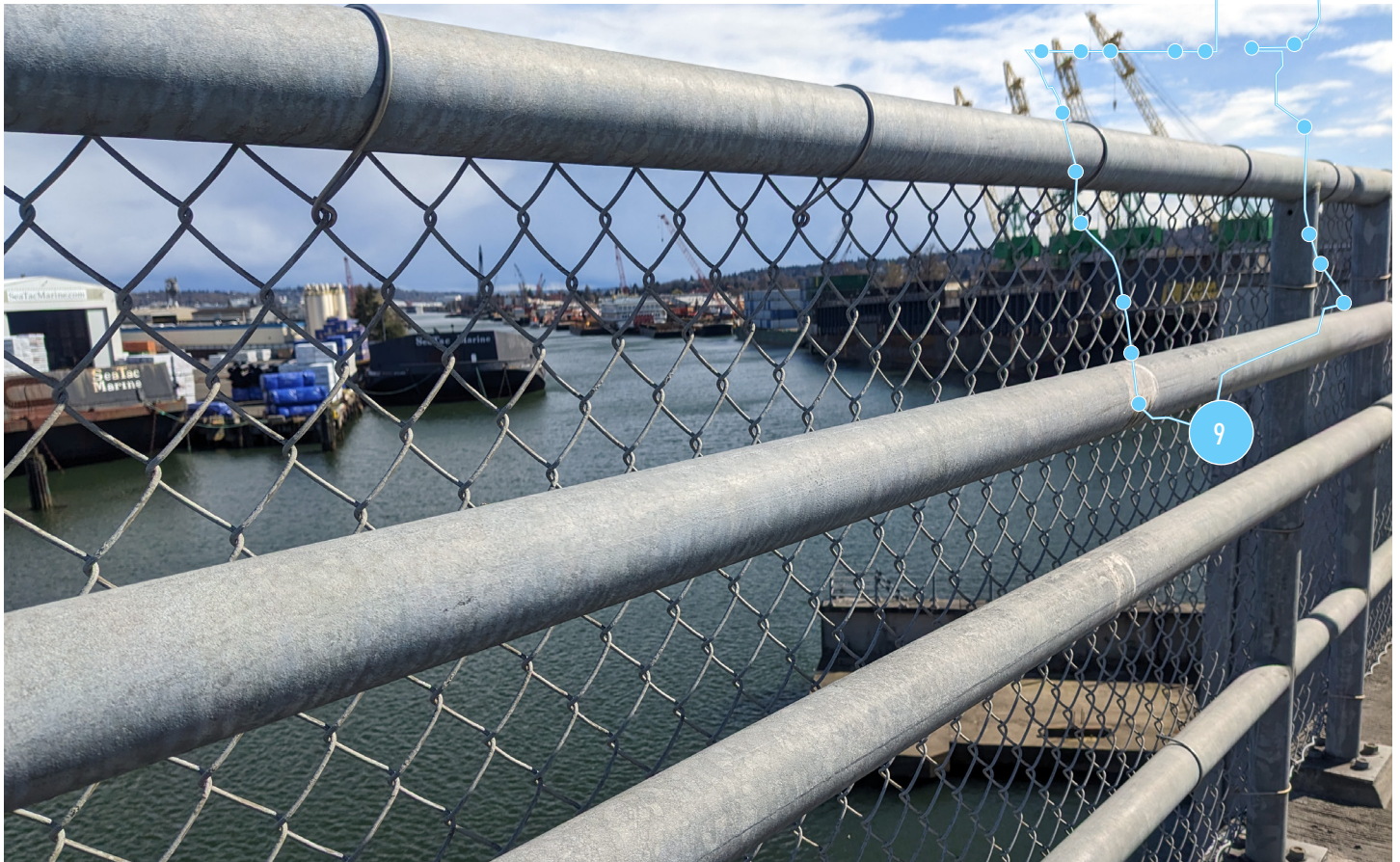
Figure 53. 1st Avenue South Bridge (Photo by author)
