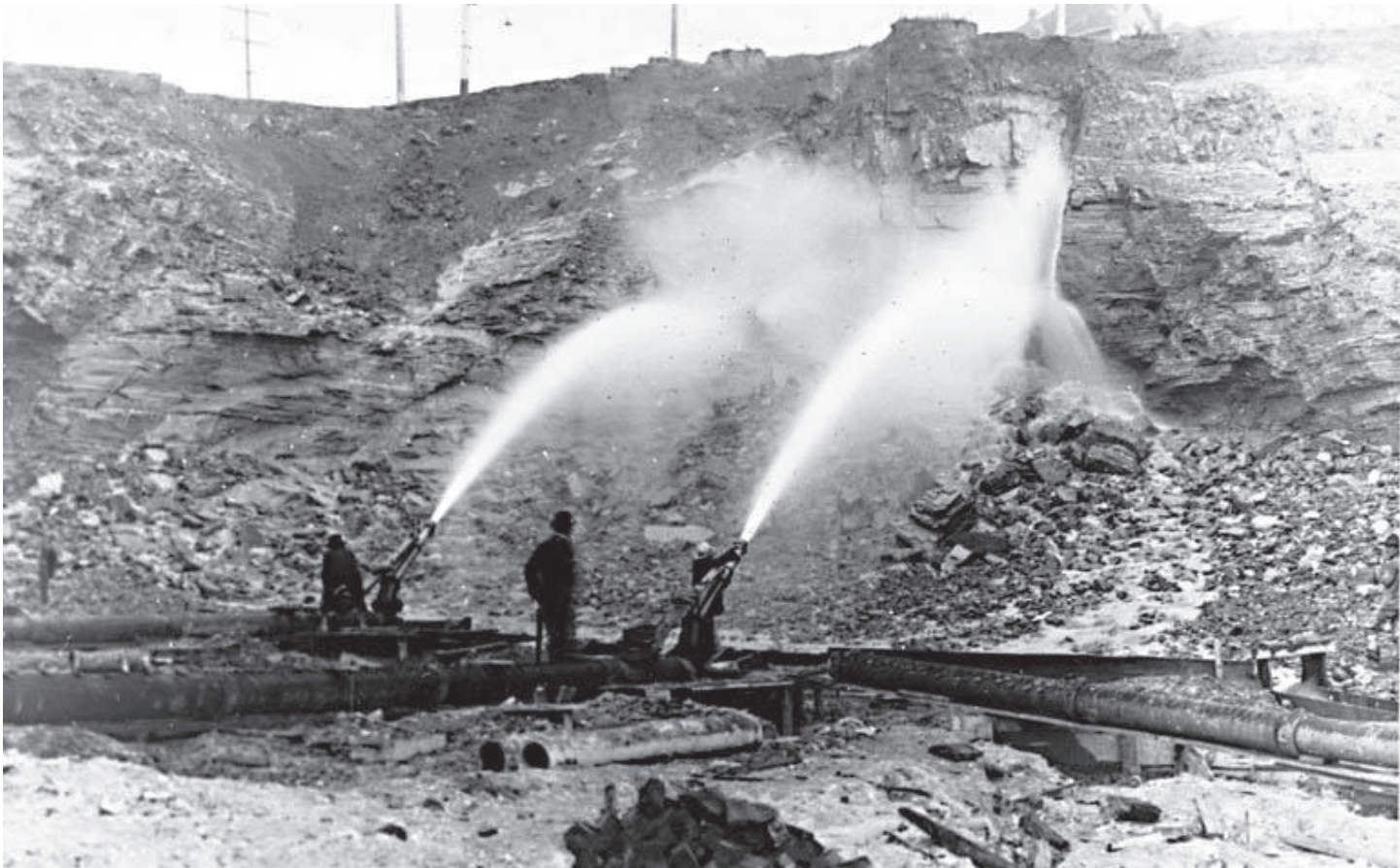
Figure 30. Semple's South Canal project showing hydraulic giants at work, ca. 1901 (University of Washington Libraries, Special Collections, UW4227)
