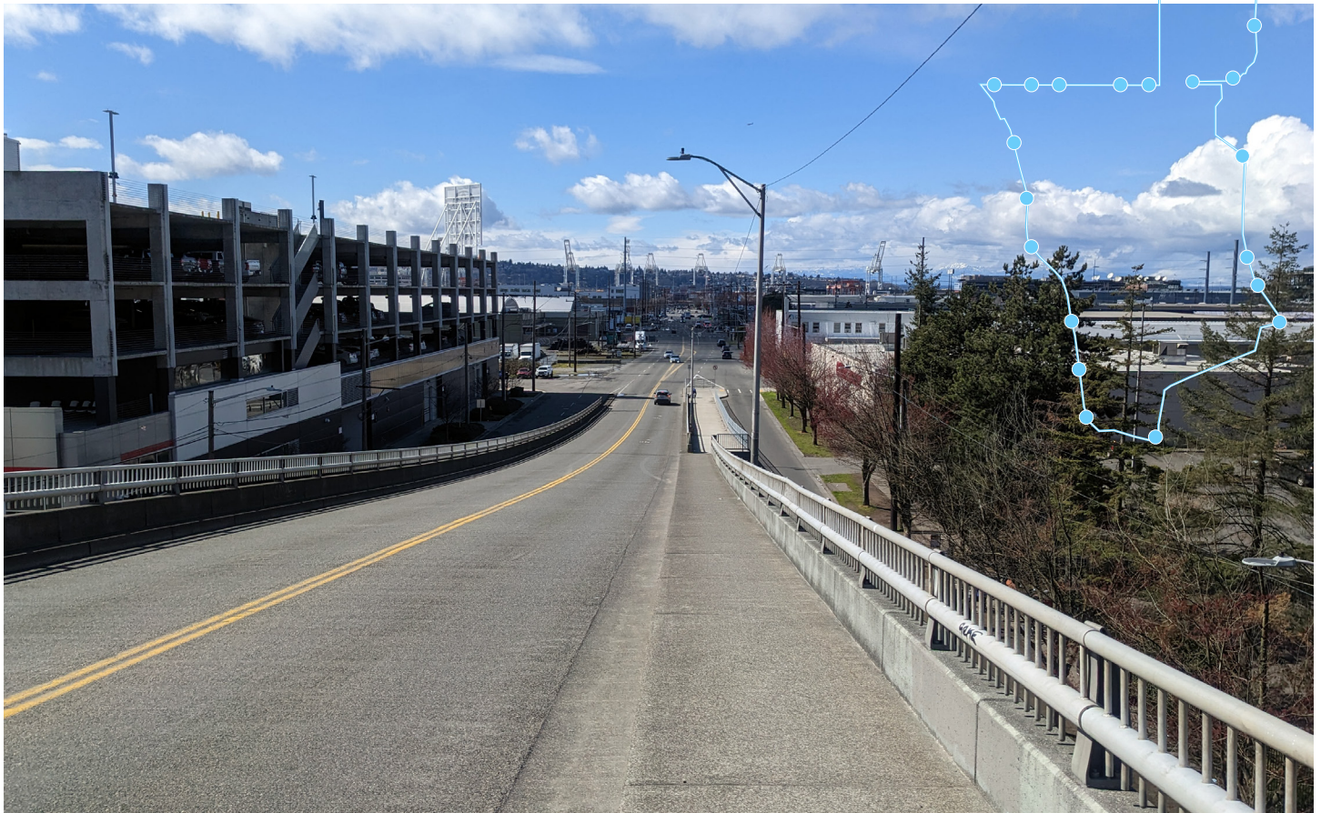
Figure 21. Site Photograph at the Holgate Street Bridge
