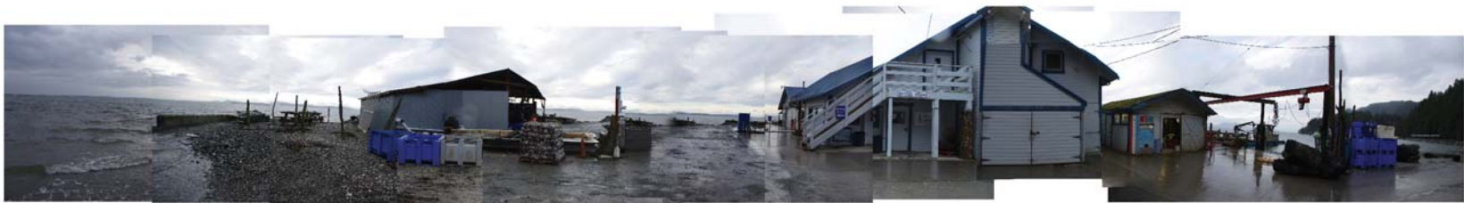
Figure 41 Existing site conditions viewing west. from left to right: storage, existing retail and dock (Author).
