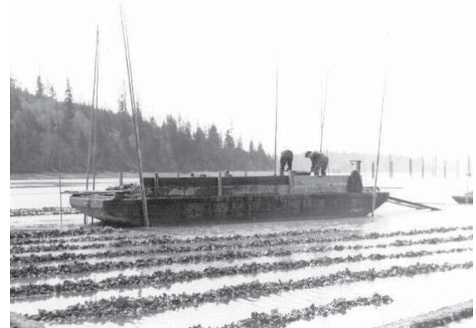
Figure 9 Digging ditches for oyster mudflats (Dewey).
