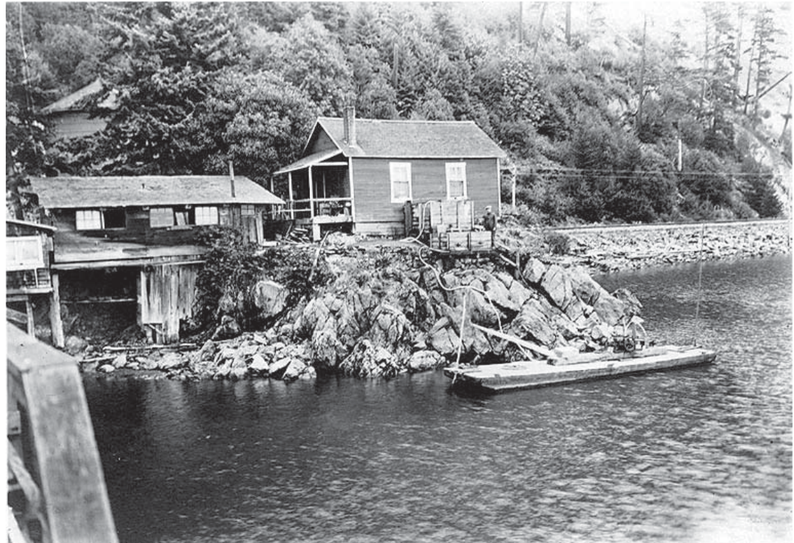
Figure 12 Building on rock outcrop was the first experimental oyster hatchery in Washington (UW Special Collections).
