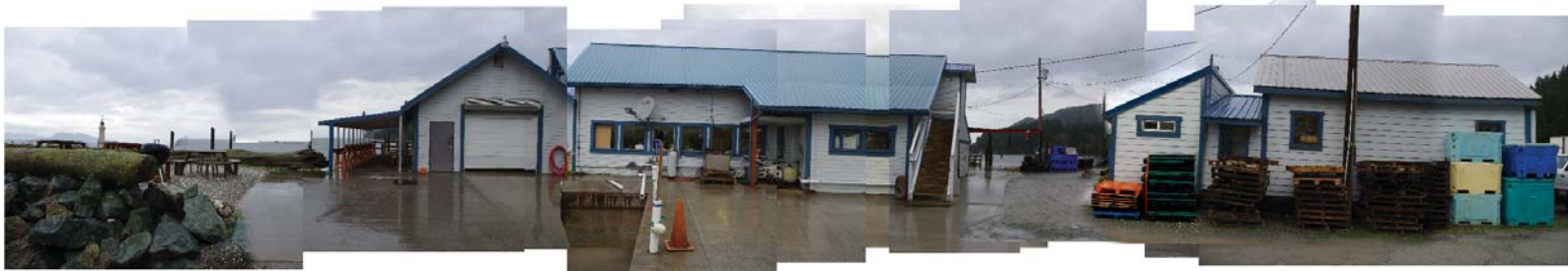
Figure 42 Existing site conditions, view towards north, from left to right exterior customer spaces, processing, retail, restrooms, and workshop (Author).
