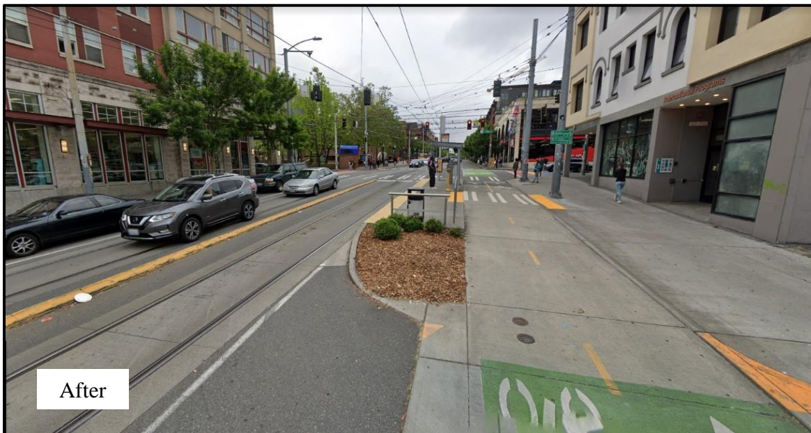
Figure 4.3.2 Broadway After Project Implementation (36)
