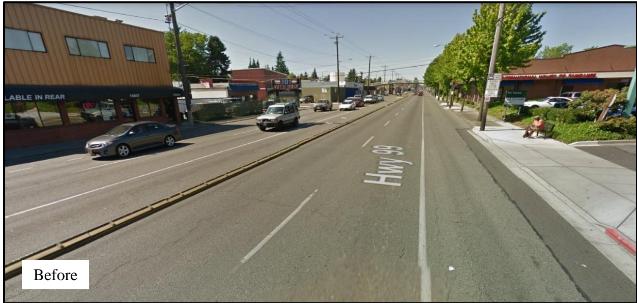
Figure 4.5.1 Aurora Ave N Before Project Implementation (36)
