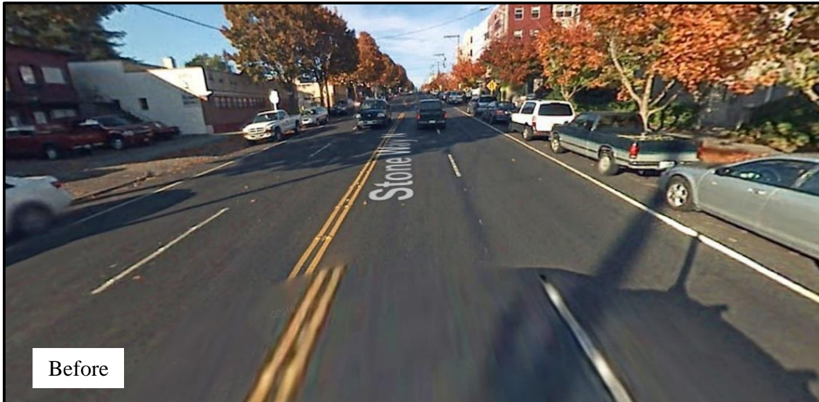
Figure 4.4.1 Stone Way N Before Project Implementation (36)
