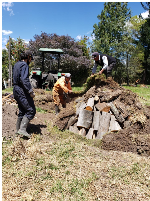
Image 44. Building a buried charcoal furnace, second attempt. Photo by author.
