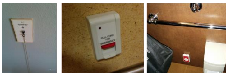
Figure 4.4. Wall sensors in 3 different communities. Two pull cords (left and middle) and a button (right)
