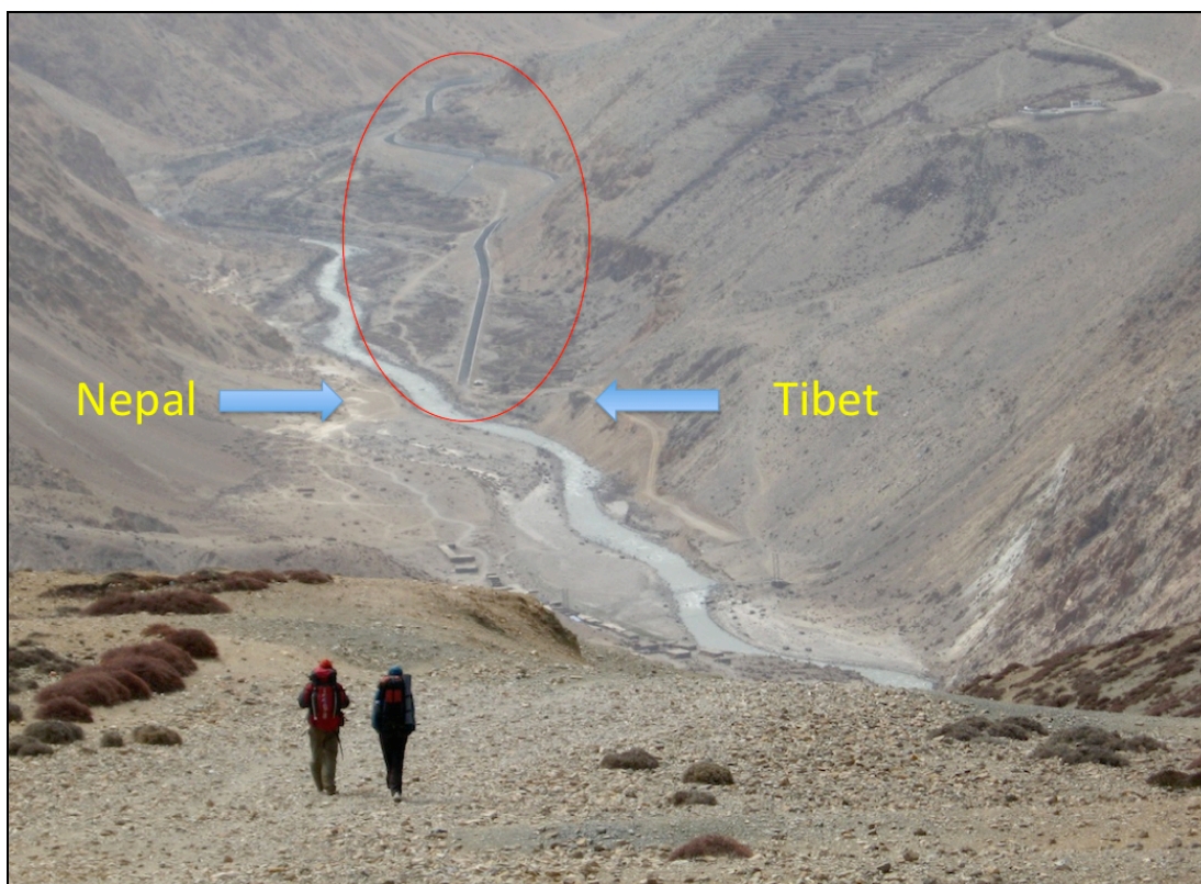
Figure 6.12 Just across Humla’s border with Tibet, a paved road was built by the Chinese government in less than three years. The WFP-supported Hilsa-Simikot road is supposed to cross the Nara La pass and join up. (Photo: Jeff Masse)
