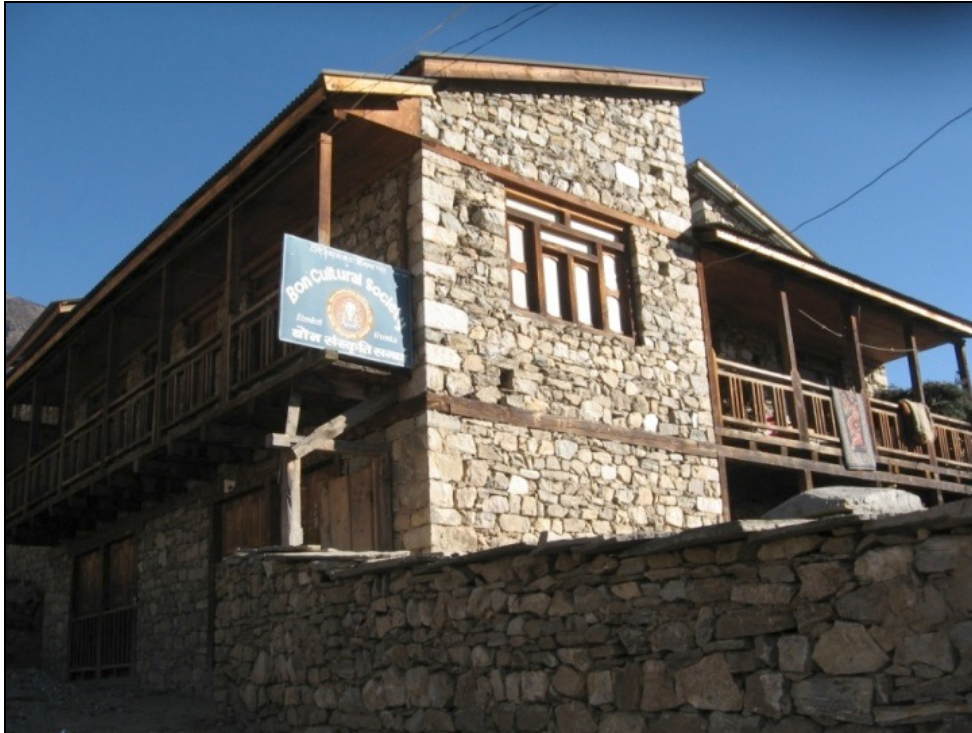
Figure 3.3 A newly constructed shared home and NGO office in Simikot.
