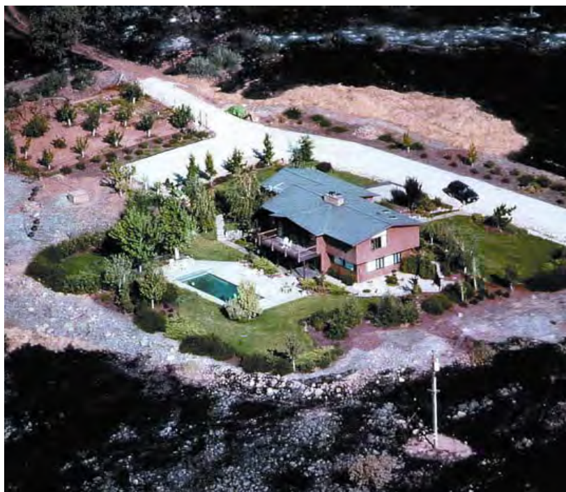
Figure 2: A Ross Valley home with a maintained defensible space that survived a wildfire (Source: Ross Valley Fire Department. Defensible Space . www.rossvalleyfire.org/ )
