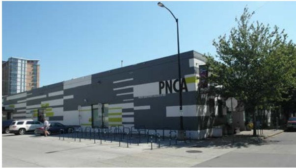
Pacific Northwest College of Art (PNCA) / Existing Building
