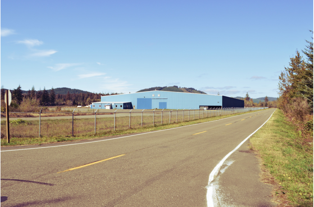
Fig 3.6: A photo of the existing warehouse from the southeast corner of the Forks Industrial Park.
