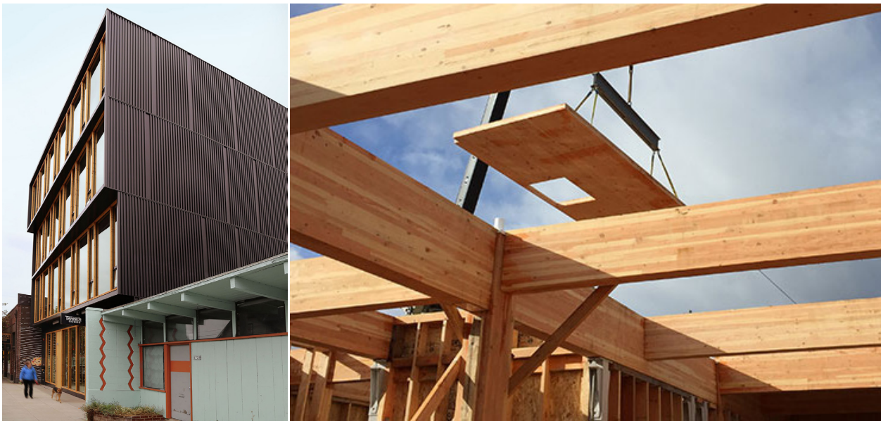
Fig 2.23: Albina Yard in Portland, OR. Building Design by Lever Architecture and Reworks Inc.
