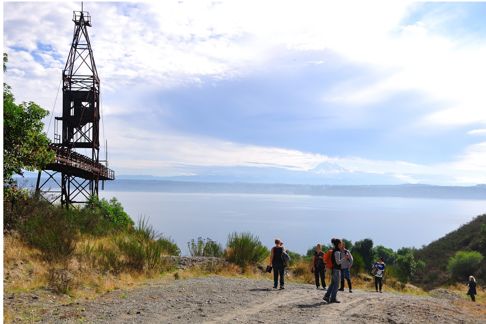
Figure 2.11 Gravel crane structure in Maury Island Gravel Mine site in 2011
