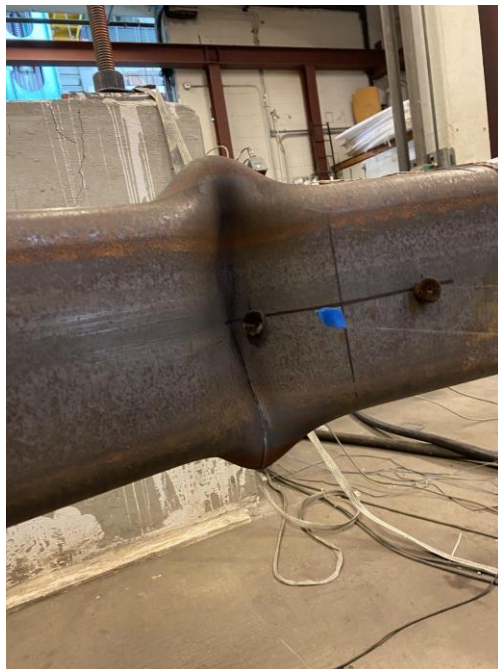
Post-Tearing cupping at Center of Specimen: 2.25" Cycle 2 C
