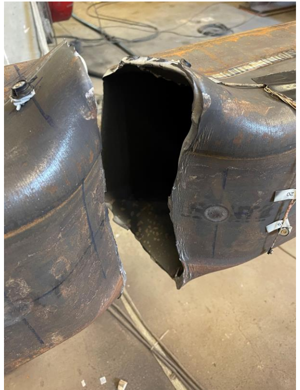
Large residual local deformations following fracture
