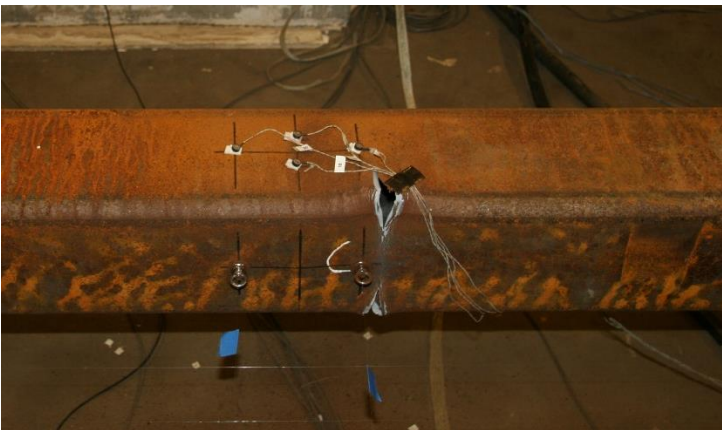
Tearing at corners on the east wall: 2.75" disp.
