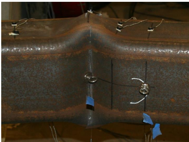
Cupping and wrinkling following tearing: cycle 18
