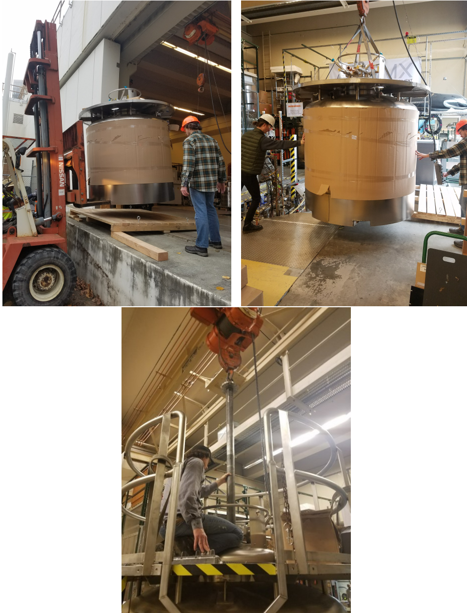
Figure 4.22: Installation of 2500 LL helium dewar.
