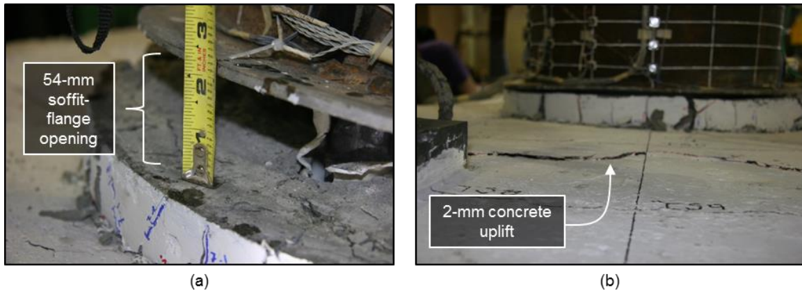
Figure 5.47: WRCUB (a) Soffit-flange opening at first bar fracture, and (b) South concrete uplift at 10.53% drift North
