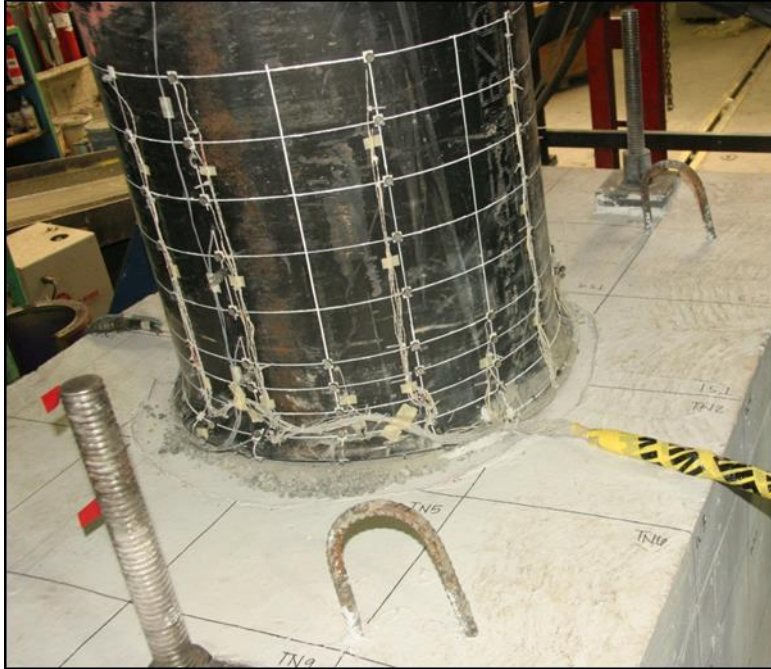
Figure 5.73: EMB96 Specimen damage at termination of test
