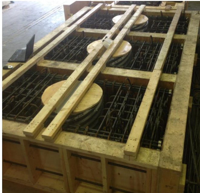
Figure 4.7: Cap Beam Reinforcing and Formwork
