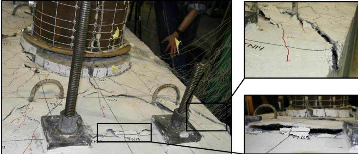
Figure 5.33: WRC North cap beam damage at 11.47% drift South
