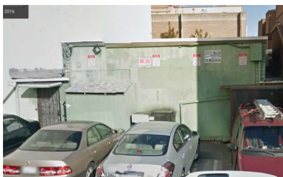
Figure 3-8. Back side of street-oriented building
