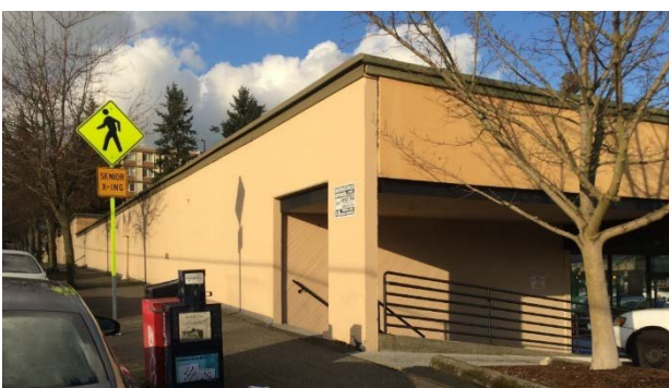
Figure 3-7. Building oriented away from street.
