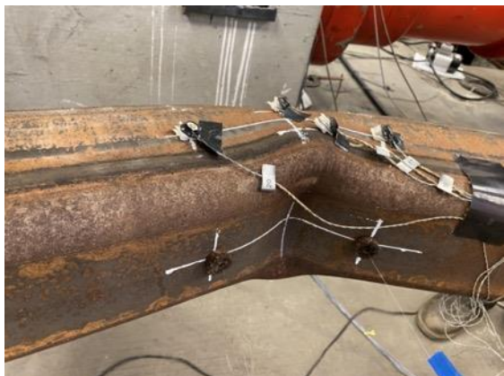
Cupping at Center of Brace: 3.75" Cycles
