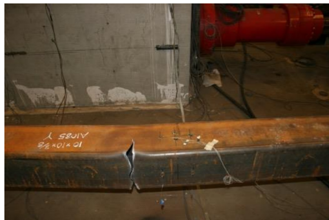
Tearing Across East Wall: 1.75" Cycle 2 T
