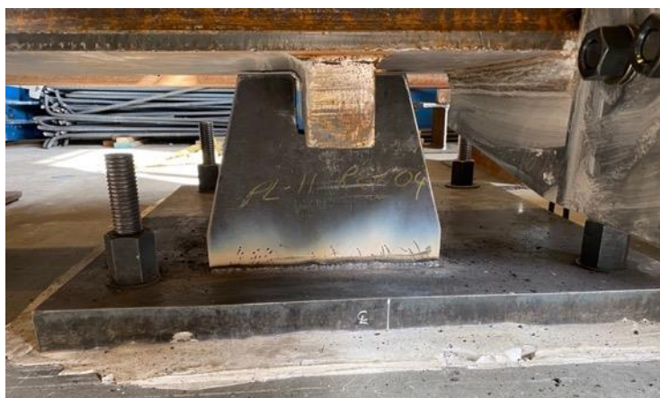
Figure 3.23. Keyway Plate Dimensions (a) and Keyway Plate Welded in Place (b)
