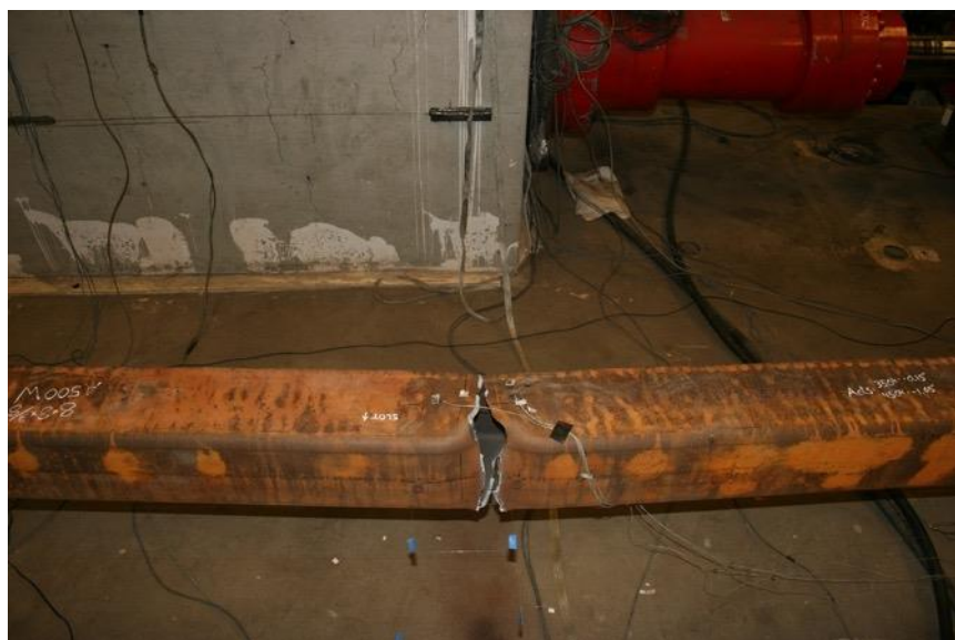
Tearing at Center Immediately Prior to Fracture: 2.25" Cycle 1 T
