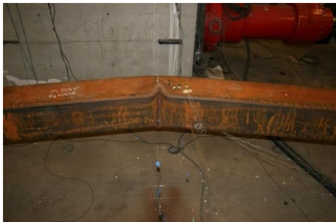
Cupping After Tearing Through Cross Section: 2.25 Cycles 1 & 2 C
