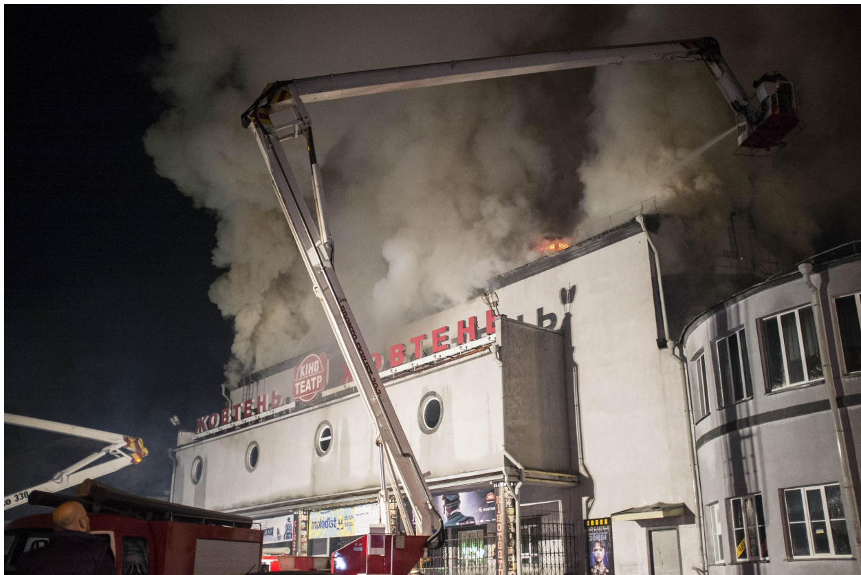
Smoke and flames billow from the roof of Zhovten Cinema on October 29, 2014. (Chris Collison)
