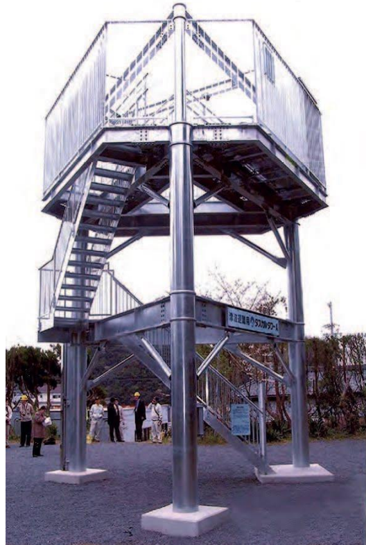
Figure 12: Photo of an evacuation tower
