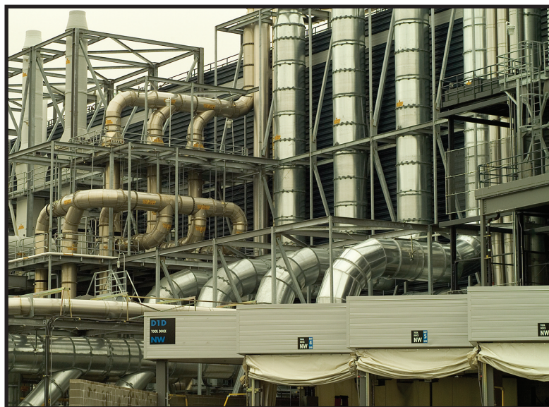
At its peak, Intel's 778,000-square-foot D1D fab employed 4,000 union construction workers. The new D1X will be twice as big. Photo by Bruce Forster Photography, Inc.
