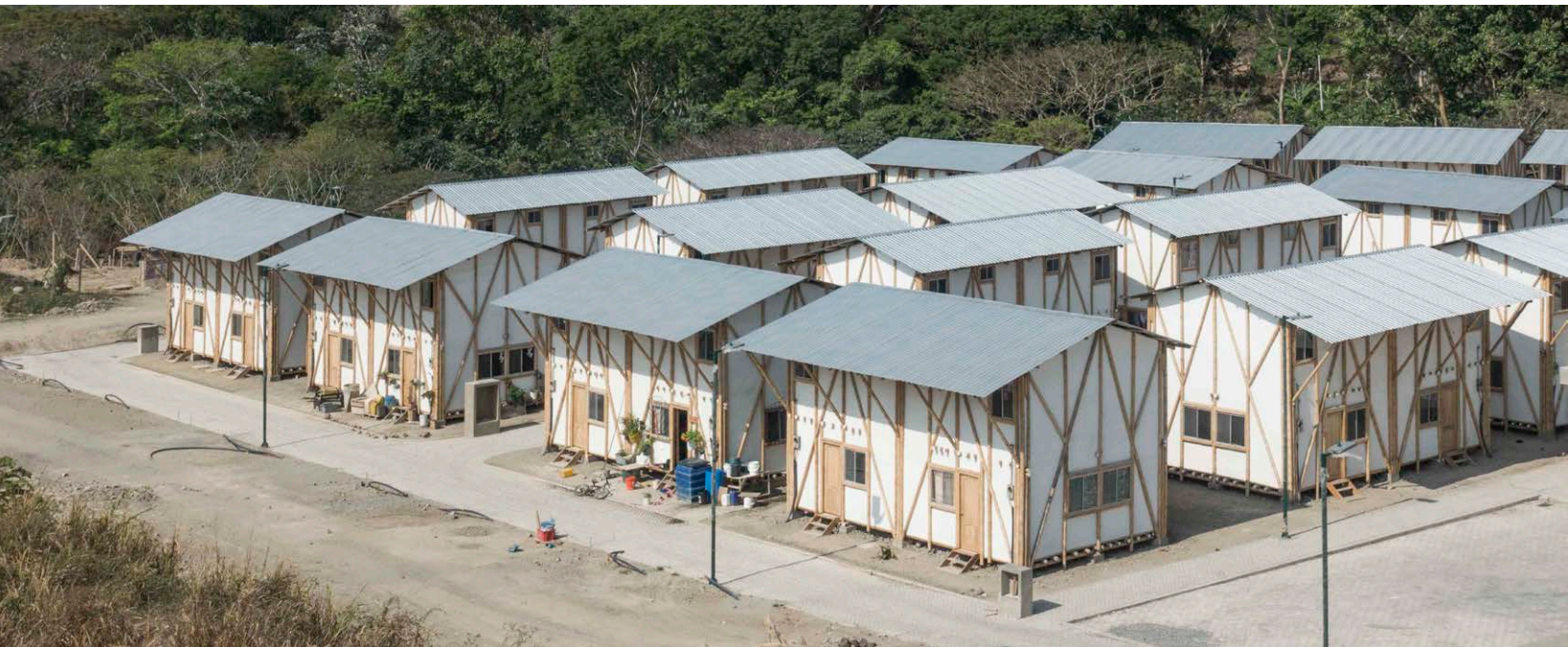
Fig B.58 - Duplex units with full services provided La Chorrera, Pedernales, Ecuador
