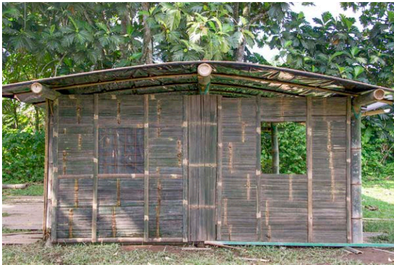
Fig 1.13- Enclosed, panelized transitional shelter
