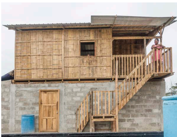
Fig 4.18 - CMU infill below modular bamboo panels, Rural context: Muisni, Ecuador
