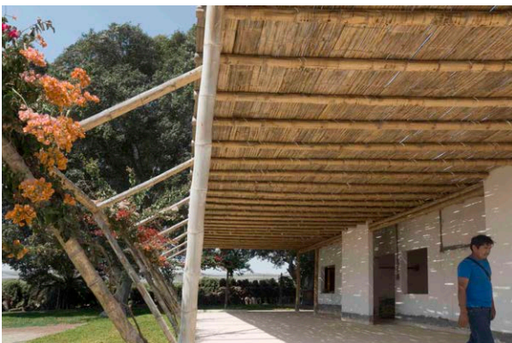
Fig 4.26 - Vineyard patio, Pisco, Peru. Contractor: Carlos Huauya Erribares
