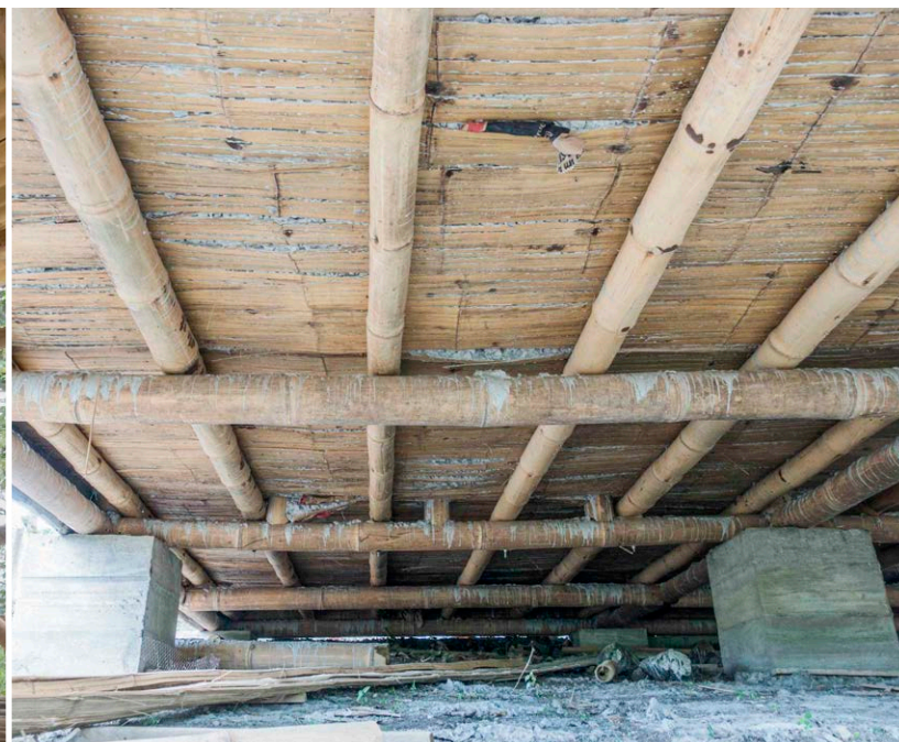
Fig B.51 - Single story bamboo housing reconstruction Jama, Ecuador. Architect: Silvia Flores
