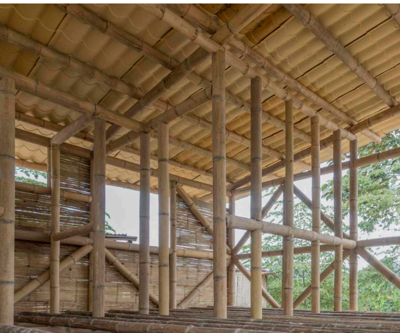
Fig B.50 - Single story bamboo housing reconstruction Jama, Ecuador. Architect: Silvia Flores
