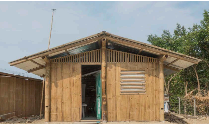
Fig B.65 - CAEMBA home, slowly being upgraded by residents outside of Esmeraldas, Ecuador
