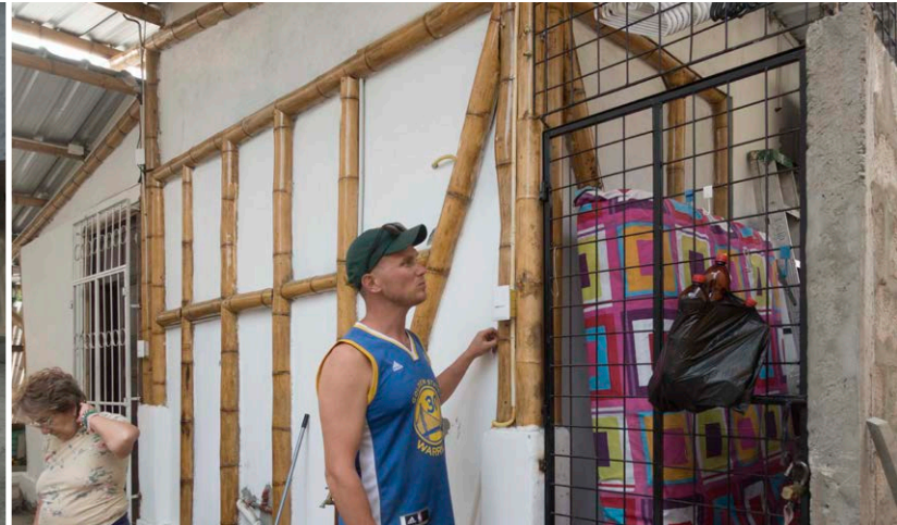
Fig B.26 - Disaster relief housing Designed and built by Bahia Beach Construction
