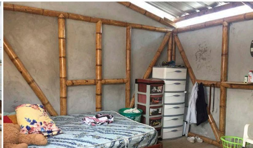
Fig B.41 - Disaster relief infill housing Designed by author with contributions by local contractors
