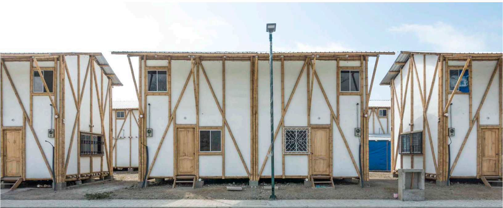
Fig B.61 - Duplex units with full services provided La Chorrera, Pedernales, Ecuador
