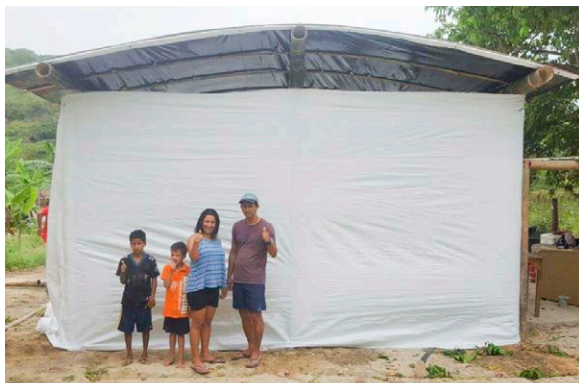
Fig D.6 - Emergency shelter with plastic privacy screen
