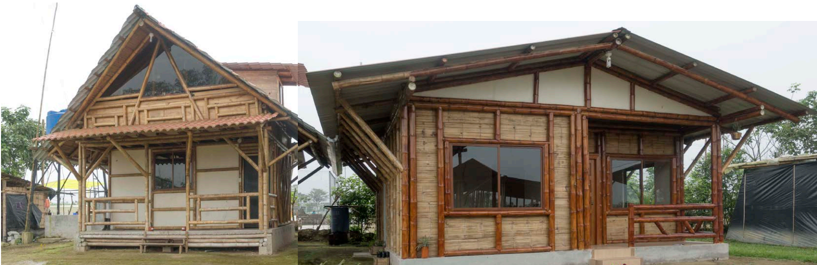
Fig B.80 - Two homes designed and built by Efrain, Near Santo Domingo, Ecuador
