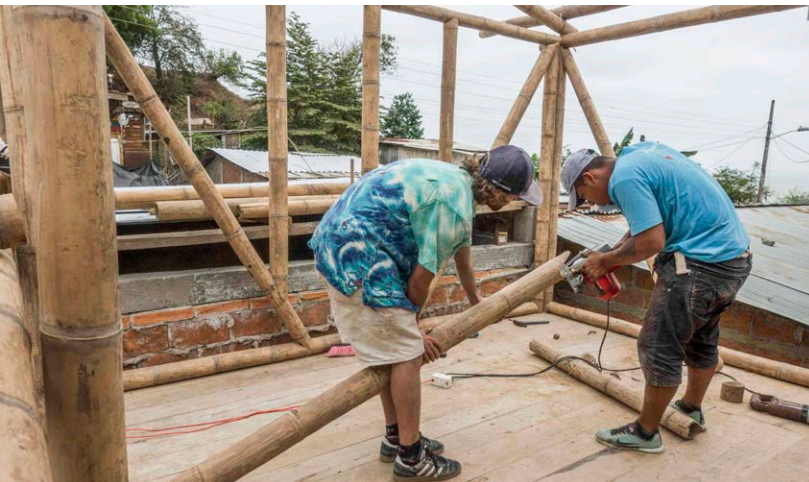
Fig B.40 - Disaster relief infill housing Designed by author with contributions by local contractors
