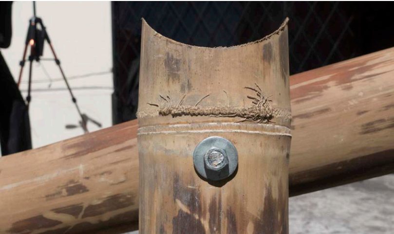
Fig B.99 - Precut and partially assembled components allowed our group to complete the project in one day
