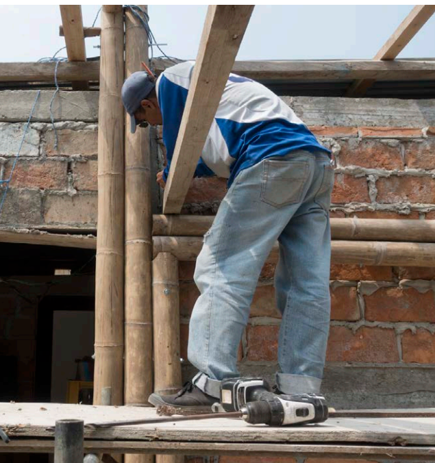
Fig B.38 - Disaster relief infill housing Designed by author with contributions by local contractors
