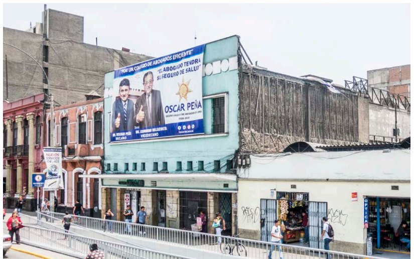
Fig 4.8 - Traditional building techniques seen through exposed quincha, Lima, Peru
