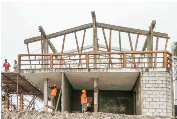
Fig 7.6 - Bamboo used to support concrete form-work
