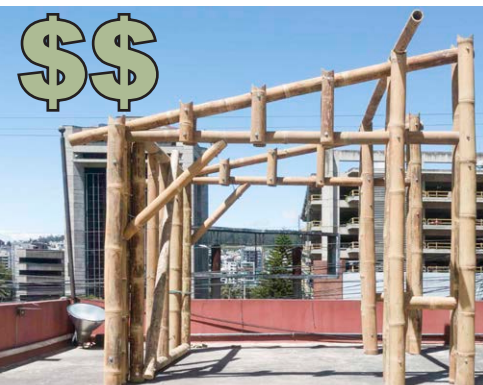
Fig 6.11 "Medium-tech" prefabrication of affordable, structural panels, Quito, Ecuador
