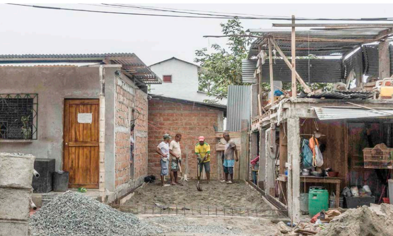
Fig B.36 - Disaster relief infill housing Designed by author with contributions by local contractors
