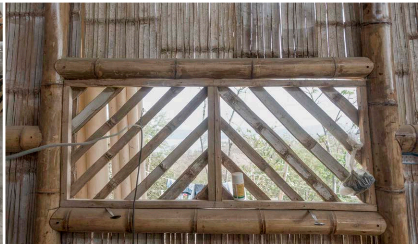
Fig B.30 - Disaster relief housing Designed and built by Bahia Beach Construction
