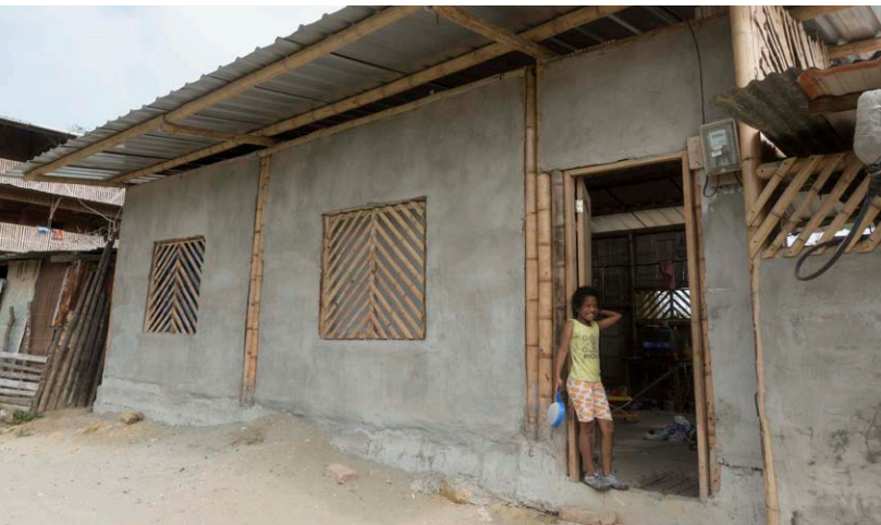
Fig B.29 - Disaster relief housing Designed and built by Bahia Beach Construction
