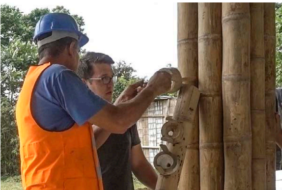
Fig 7.4 Contractor showing measuring tools made to increase speed and accuracy on the job site
