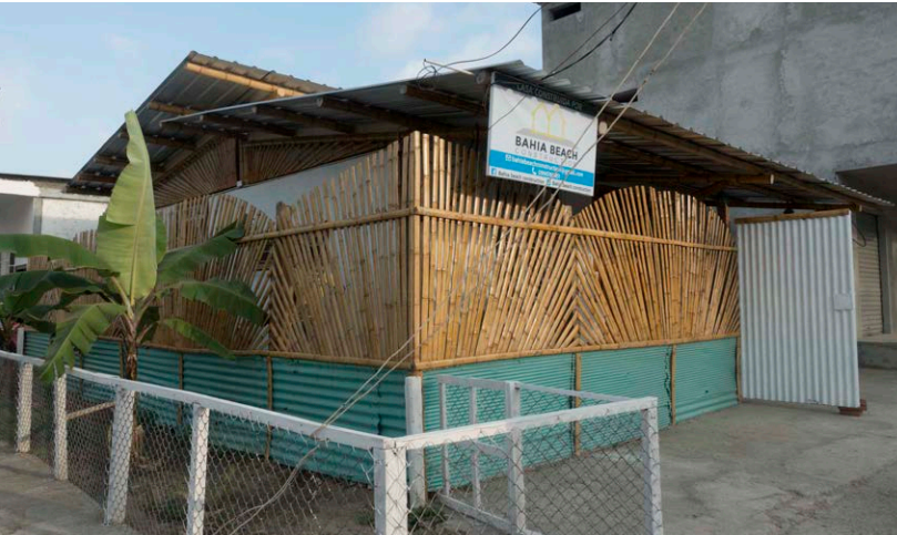
Fig B.25 - Disaster relief housing Designed and built by Bahia Beach Construction
