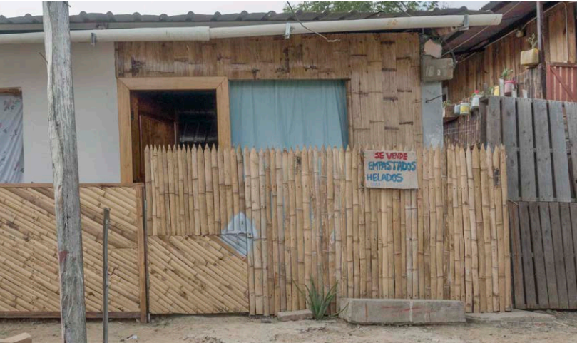
Fig B.33 - Disaster relief housing Designed and built by Bahia Beach Construction
