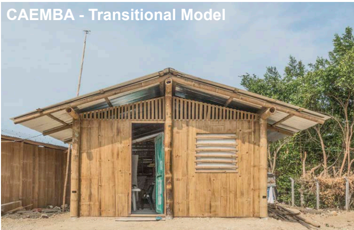
Fig 5.9 - Transitional bamboo housing, Manuel Palleres, Tonsupa, Ecuador
