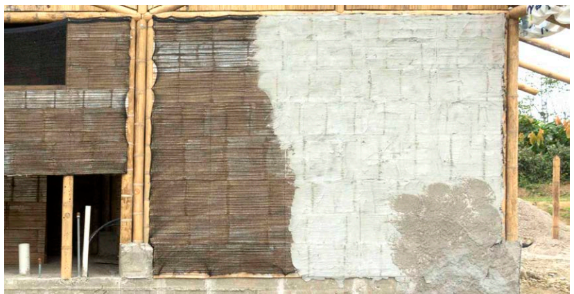
Fig 4.12 - Bahareque in process, mesh improves adherence of concrete to board. Santo Domingo, Ecuador, 2017
