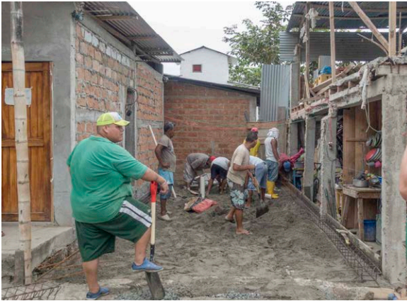
Fig 1.4 - Informal builders = cheaper construction costs
