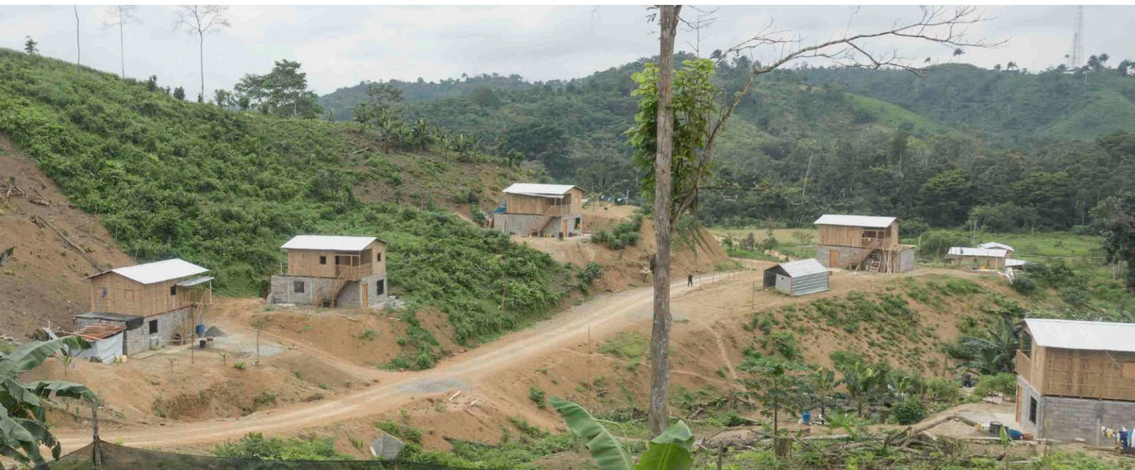
Fig B.64 - Hybrid housing development, rural greenfield site, Muisne, Ecuador
