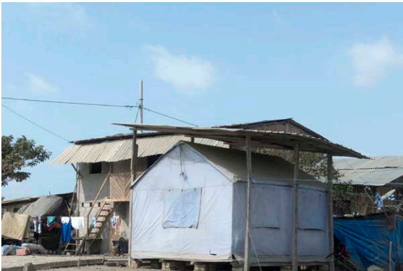
Fig D.17 - Living in emergency shelter, 18 months later
