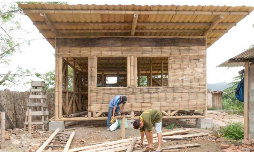
Fig B.44 - Single story bamboo housing reconstruction Jama, Ecuador. Architect: Silvia Flores
