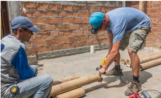
Fig 5.28 - Bahia Beach Construction: Lucas Oshun has purchased property to grow the culms used by crew (See Appendix B, #11a)
