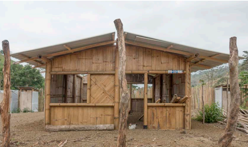
Fig B.52 - CAEMBA home, slowly being upgraded by residents outside of Jama, Ecuador
