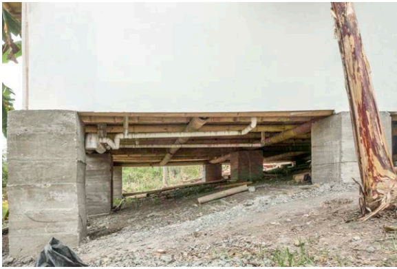
Fig 5.4 - Services included, elevated off ground Architect Silvia Flores. Jama, Ecuador
