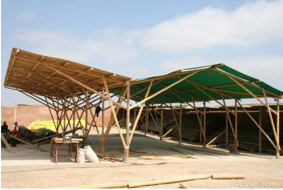
Fig D.11 - The Bamboo Training Center of San Clemente
