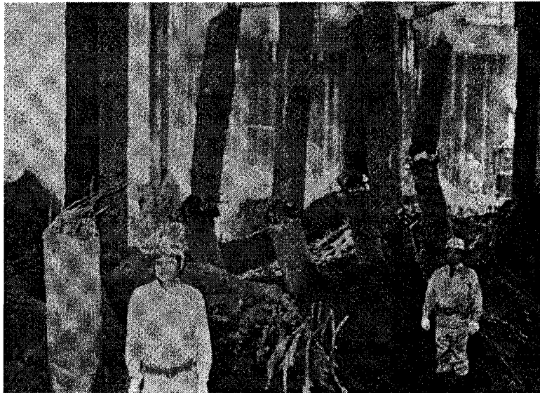
Figure 2-3 NHK Building, Japan (Hamada, 1992).
