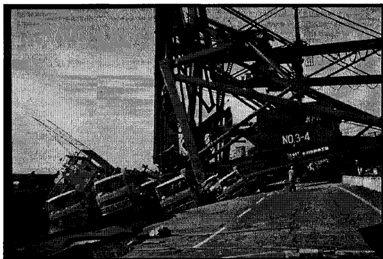
Figure 2-9 Port Island, Japan (Steinbrugge Collection).
