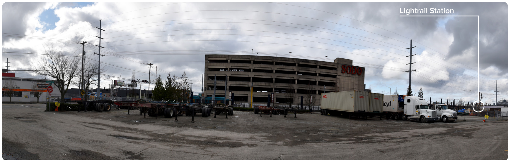
Figure 6.7: Site Photo looking West from Bisecting Alleyway
