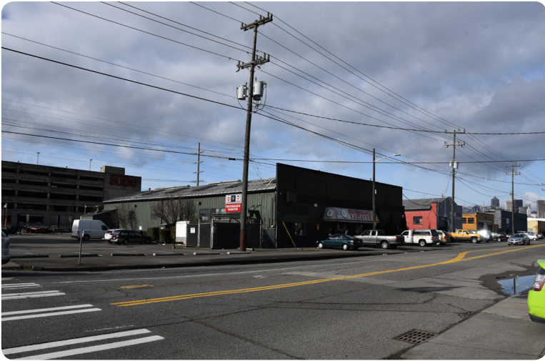
Figure 6.5: Site Photo from South East
