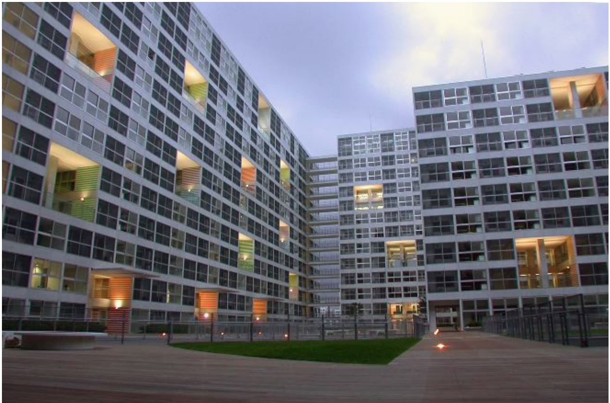
Figure 042: Shinonome Canal Court Apartments: Court yard interior
