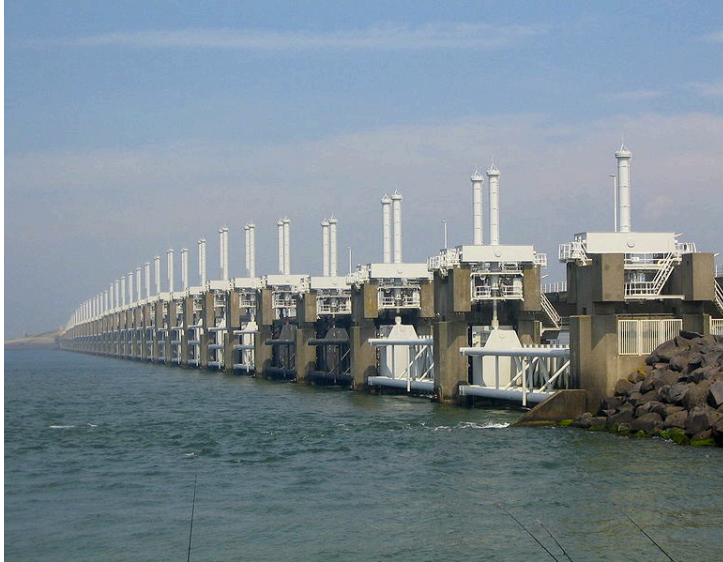
Figure 019: Eastern Scheldt Barrier, Netherlands
