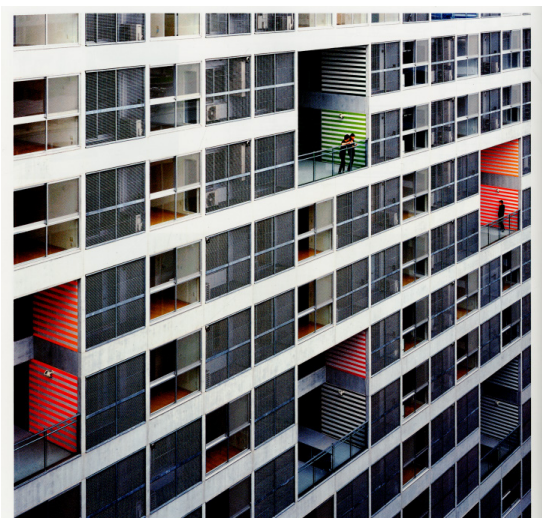
Figure 050/051: Shinonome Housing: Interior connections
