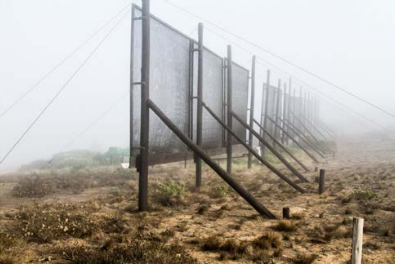
Fig 2.5: Fog-catching nets in Peña Blanca, Chile, harvesting atmospheric moisture from the Camanchaca fog. Since 2005, the system has been used to support native vegetation and provide an alternative water source in the Atacama Desert region. Source: Nick Lavars, "How Chile's Fogcatchers Are Bringing Water to the Driest Desert on Earth," New Atlas, 25 Aug. 2015
