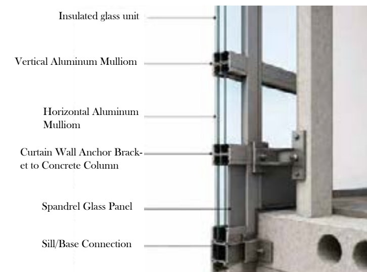
Fig 3.3: Curtain wall typycal section detail
