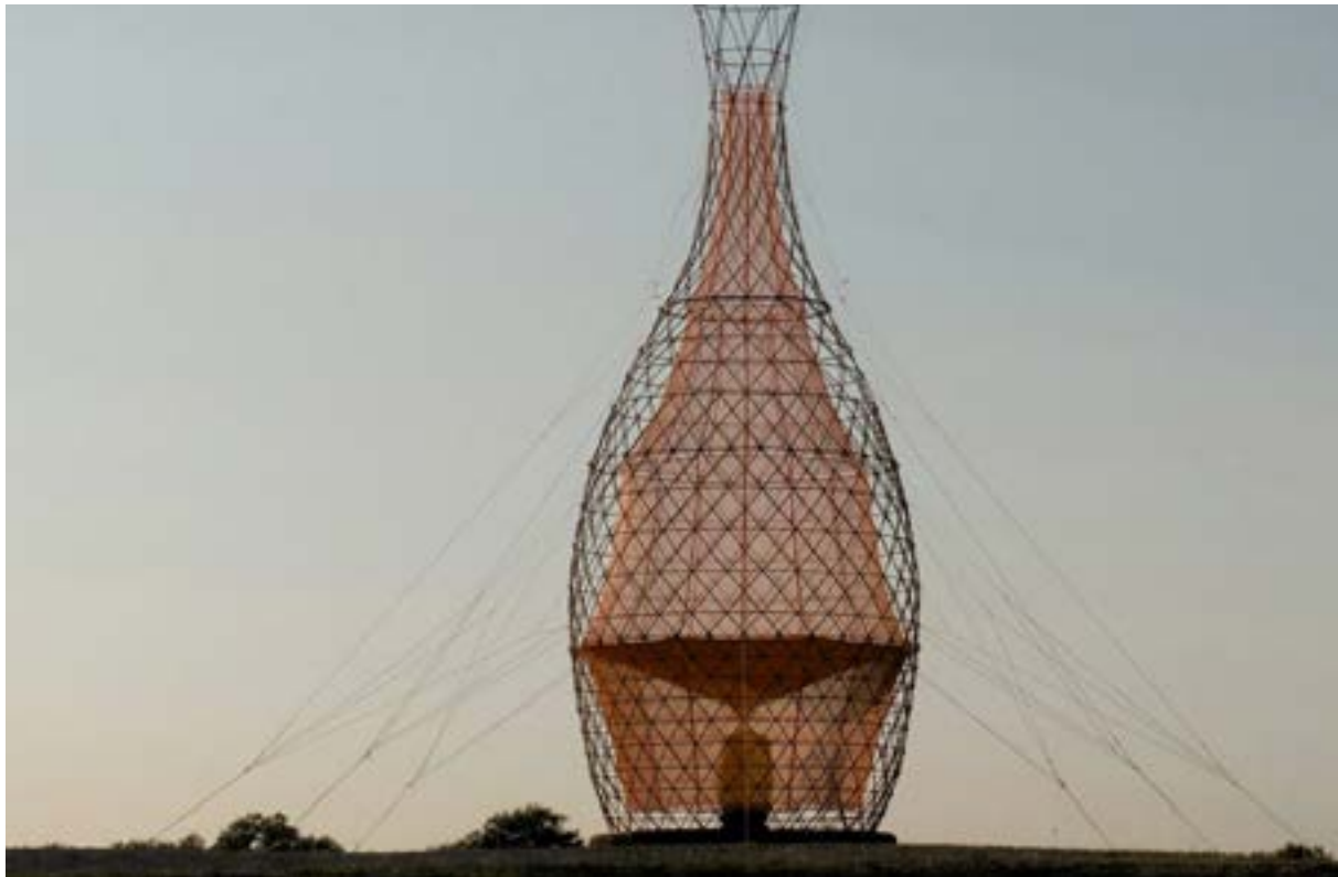
Fig 2.11: Warka Water tower. Source: Arturo Vittori, Warka Water Project.
