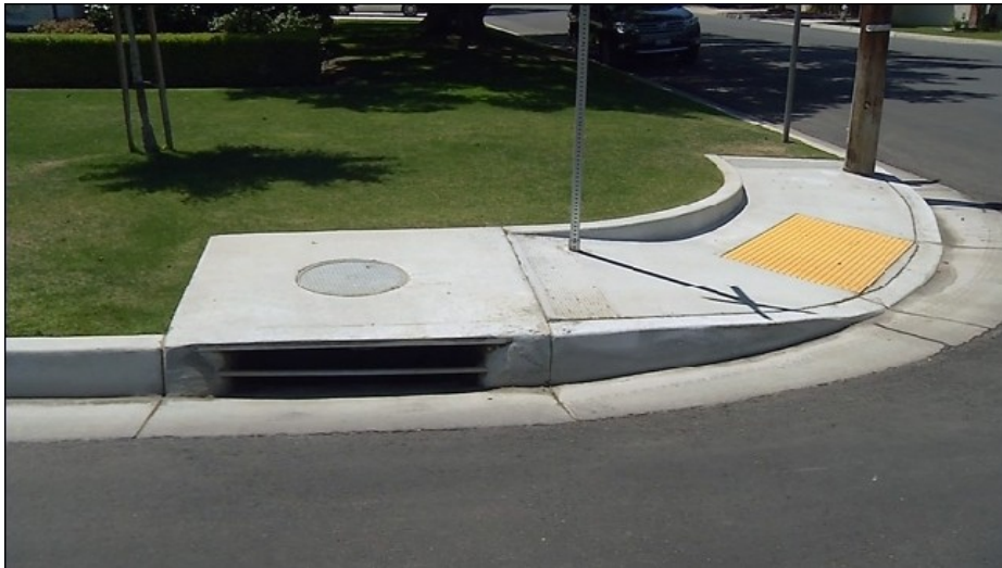
Figure 2: Curb drainage and associated disconnected, but required, ADA improvements completed in Bakersfield, CA (Ferguson, 2014)
