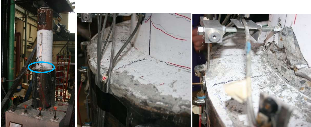
Figure 4.104. Specimen 30-21-LD a) Concrete Damage at the Edge of the Pile and b) Concrete Damage Near Base of the Column at 2.4% Drift
