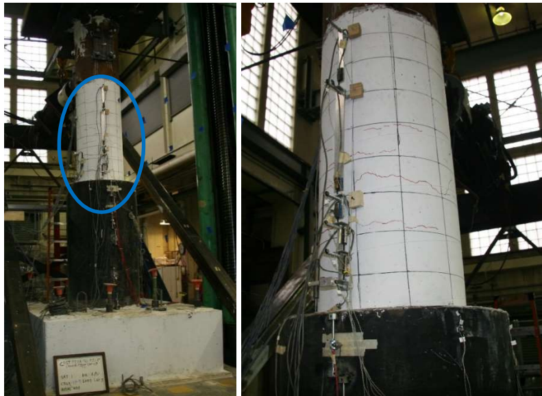
Figure 4.10. Specimen 30-21 Horizontal Cracks on North Column Face
