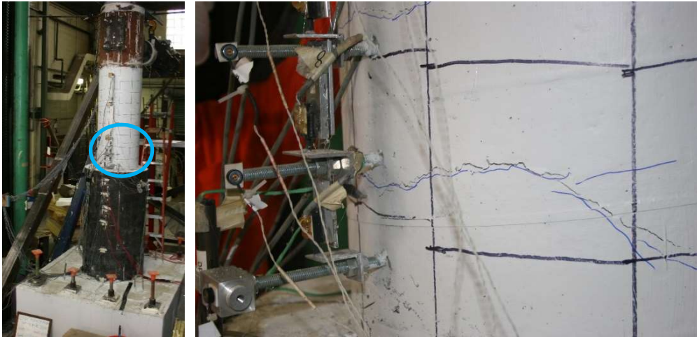
Figure 4.73. Specimen 30-21-R Column Northern Face crack at 1.75% Drift
