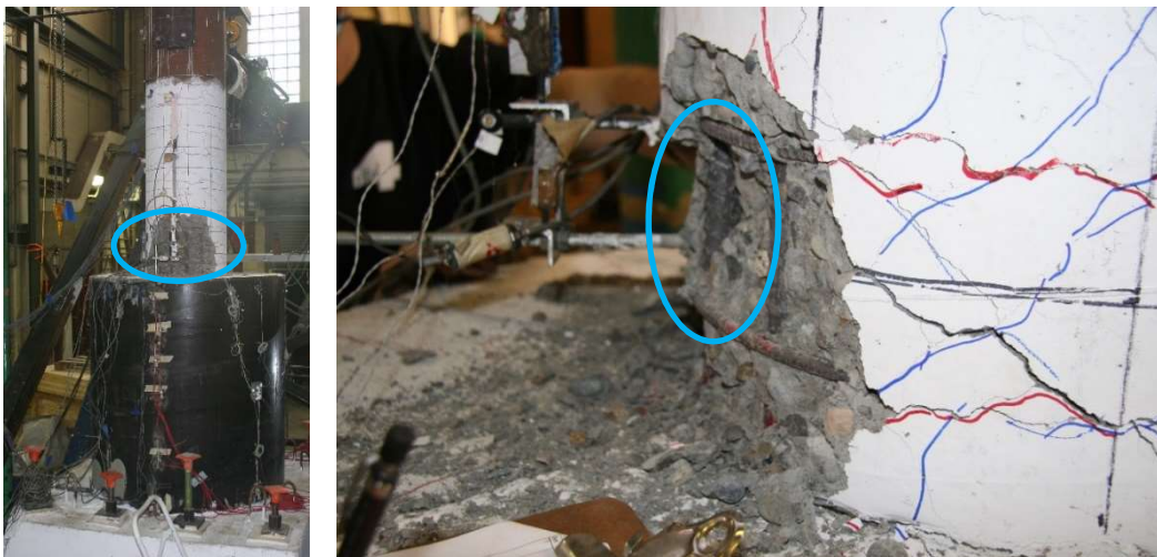
Figure 4.54. Specimen 48-21 Buckled Longitudinal Reinforcement at 5.8% Drift
