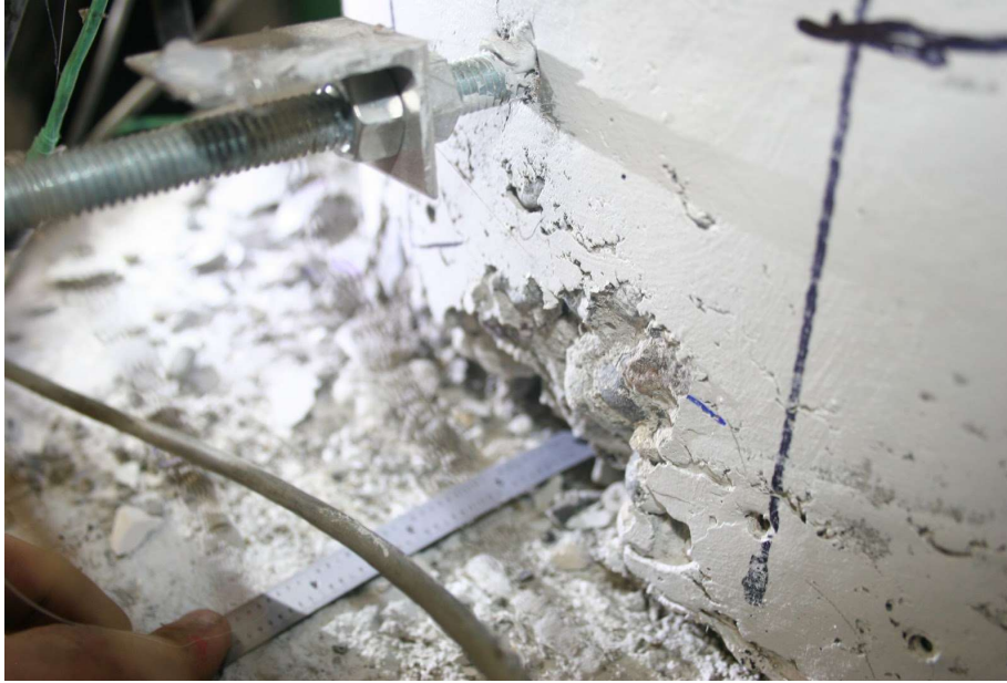
Figure 4.80. Specimen 30-21-R 2 in. Deep Crack at Northern Base of Column at 4.0% Drift
