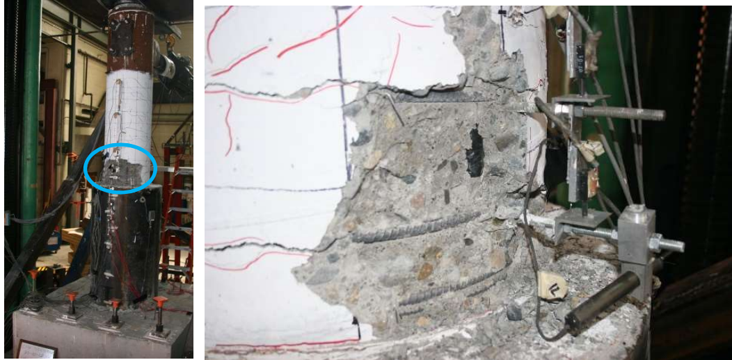
Figure 4.109. Specimen 30-21-LD Exposed Longitudinal Reinforcement at 5.5% Drift
