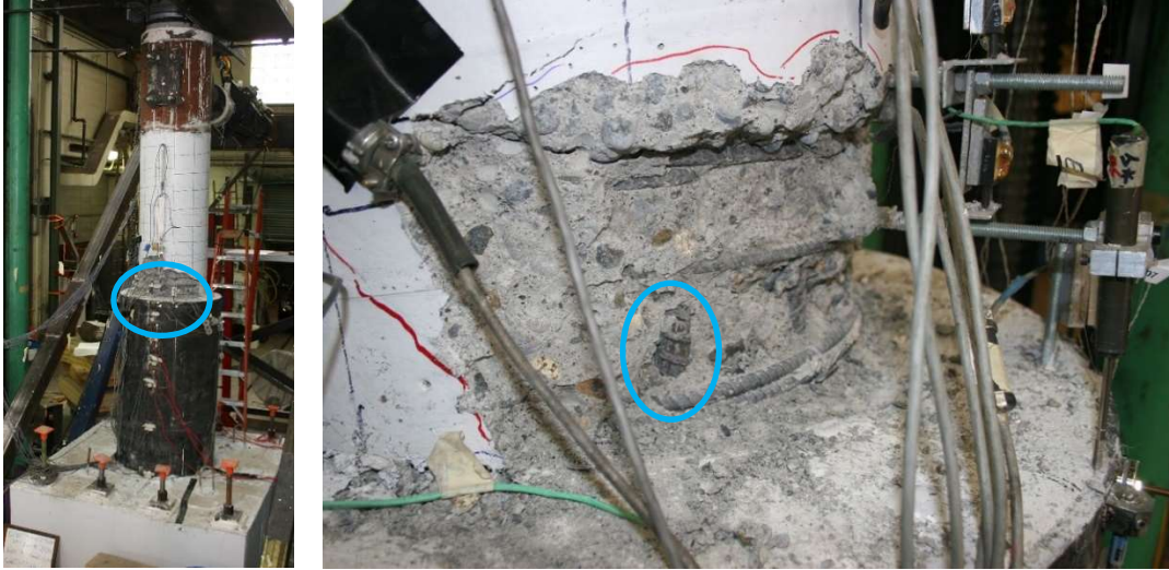
Figure 4.83. Specimen 30-21-R Exposed Northern Longitudinal Reinforcement at 5.5% Drift
