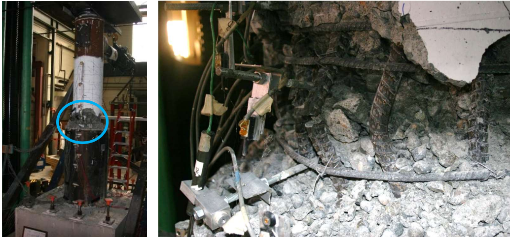
Figure 4.120. Specimen 30-21-LD Final State of Column after 9.9% Drift
