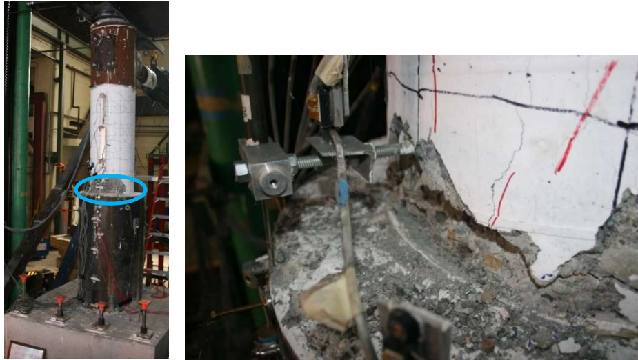
Figure 4.106. Specimen 30-21-LD Northern Column Face Spalled Region at 3.8% Drift
