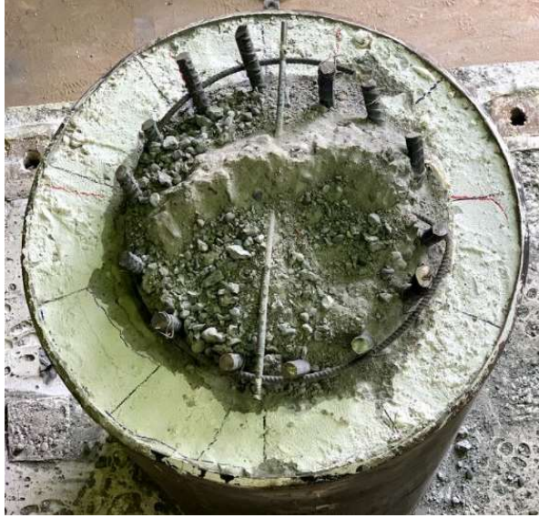
Figure 4.31. Top of Specimen 30-21 Pile with Column Removed
