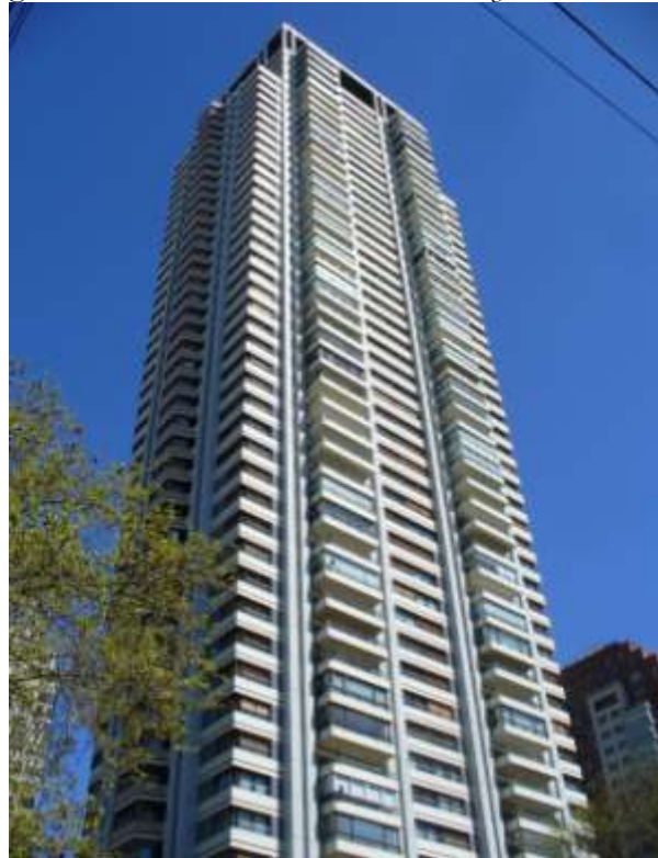
Figure Ten: Le Parc Tower, Photo Taken by Garrett Strain
