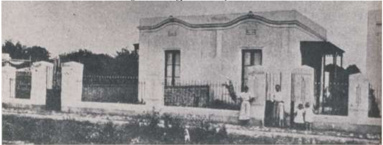
Figure Six: A Typical Casa Baja in the Suburbs
