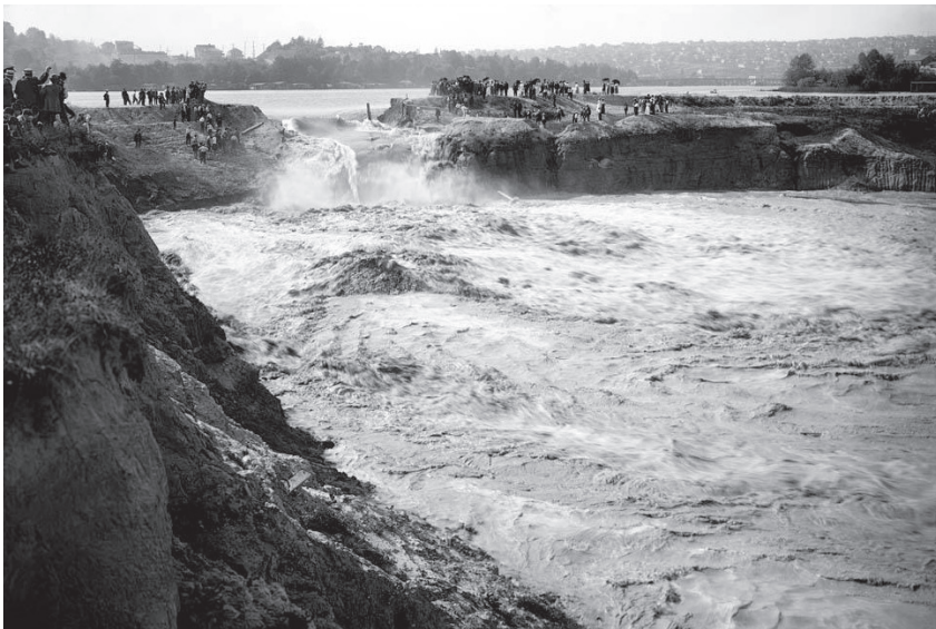
Coffer dam to Lake Union is removed, 1916
