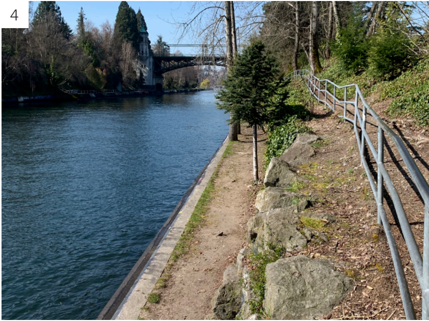
Desire paths along the terraces of the Montlake Cut with ad hoc railing
