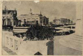
View from Manufacturers' Building across Cascades and Geyser Basin. All buildings completed.
