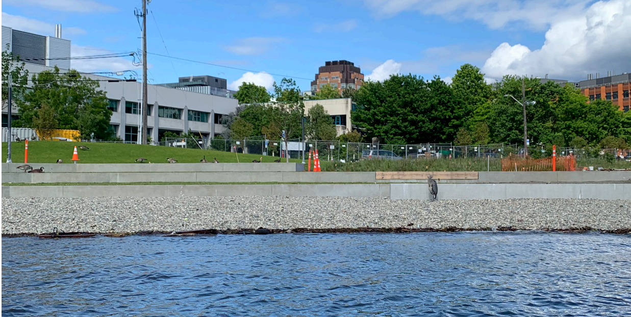
New Portage Bay Park shoreline in progress
