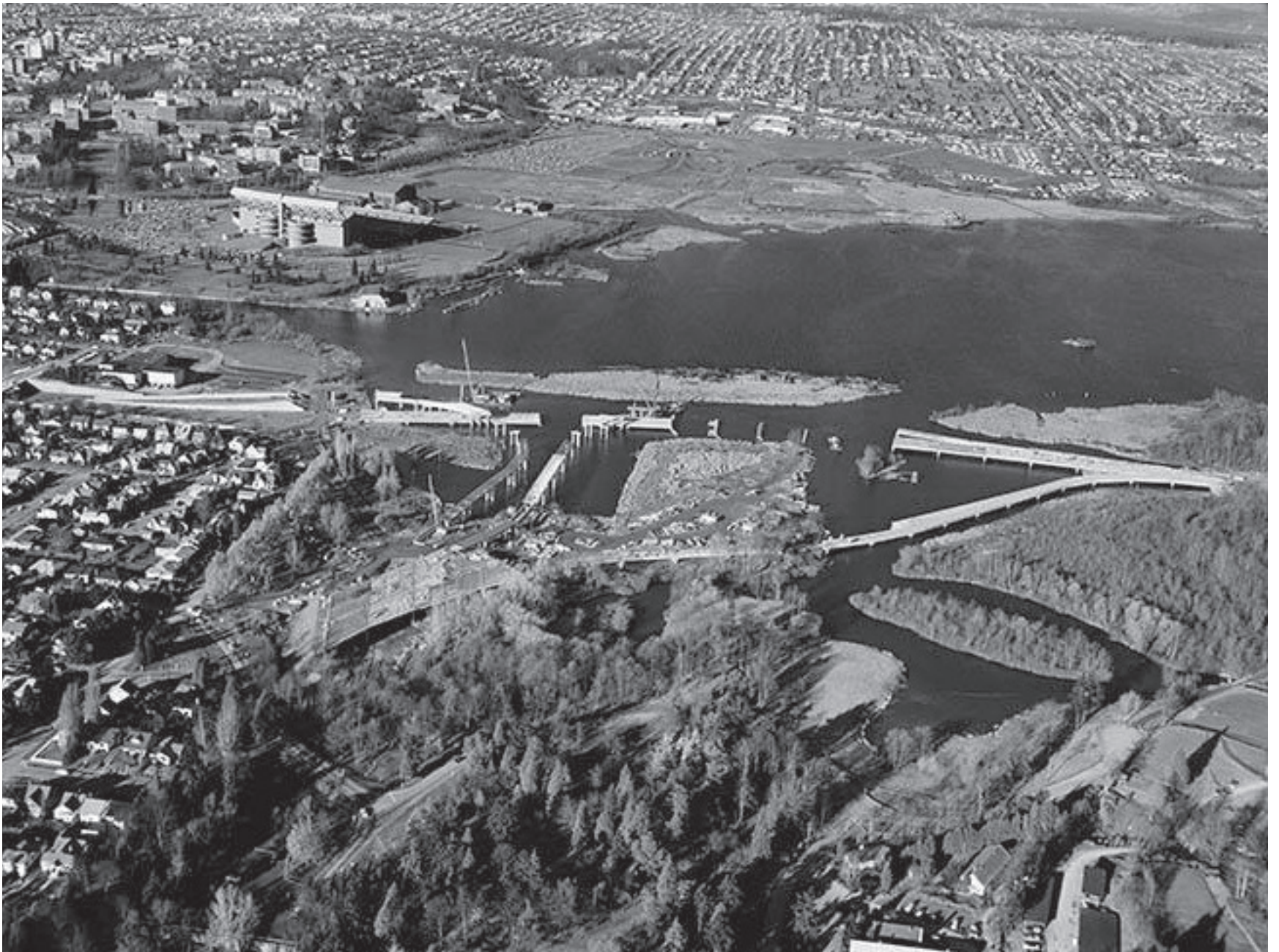
Construction of the Evergreen Point Floating Bridge in Union Bay, 1962 Museum of History & Industry, Seattle (MOHAI), John Vallentyne Photographs, 2009.23.101
