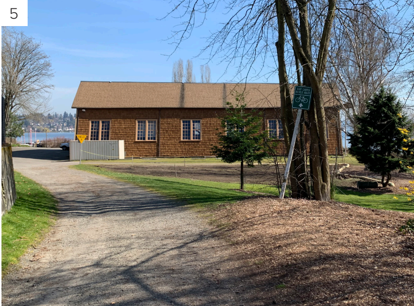
Trails become a gravel road along the underutilized area west of the Shell House
