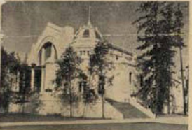
End View of Manufacturers' Building. Completed in July, 1908.
