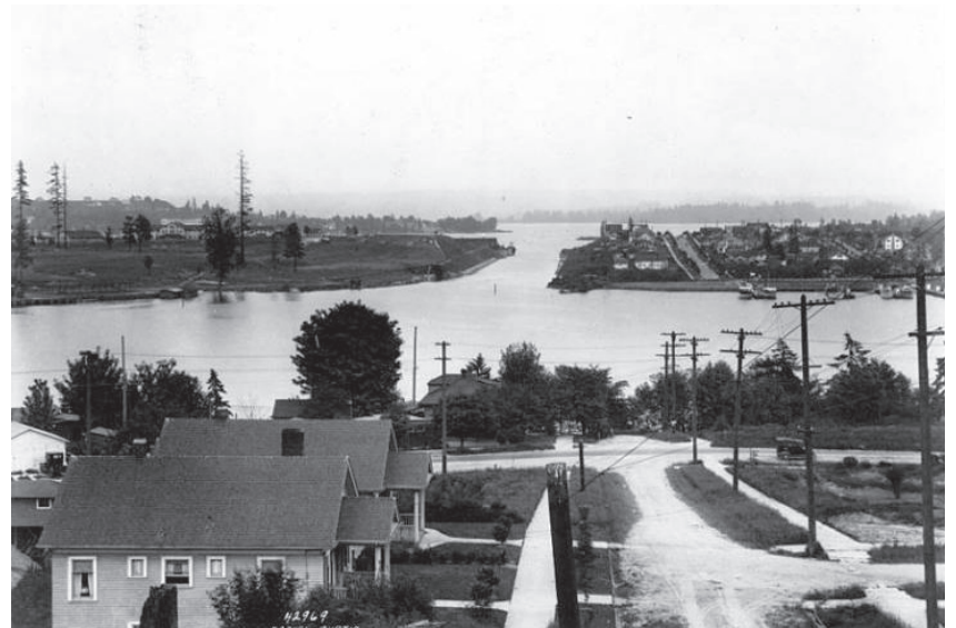
Looking east at the completed Montlake Cut with lake levels even, 1922
