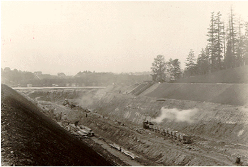
Excavating the canal, 1913
