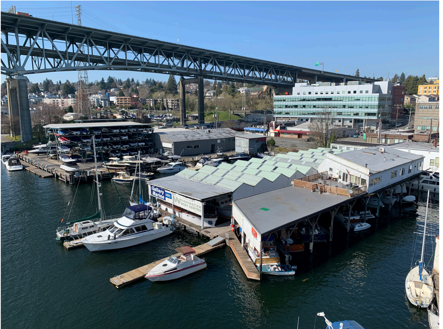
The challenge through the Lake Washington ship canal is not only bulkheads, but extensive overwater structures
