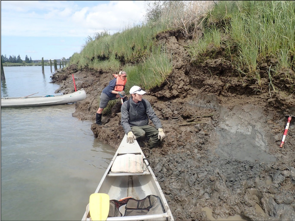
Figure 4.5 A 1-m diameter liquefaction vent along the Snohomish River. Visible on the horizon is an I-5 bridge. Other similar features surround the I-5 bridge abutments, as well as those of other area bridges.
