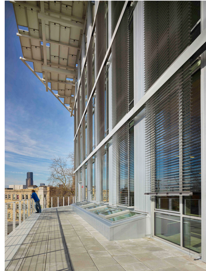
Fig. 16: Bullitt Center Facade Treatment
