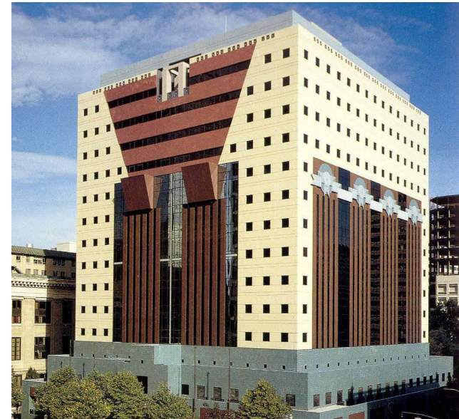
Fig. 7: Portland Public Service Building
