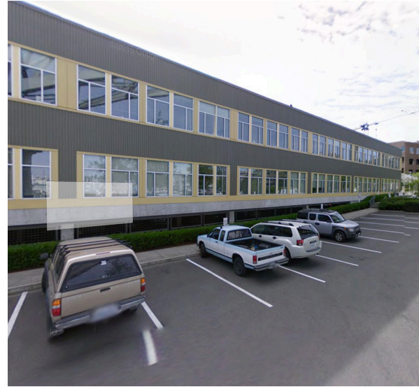
Fig. 26: Site Existing West Facade
